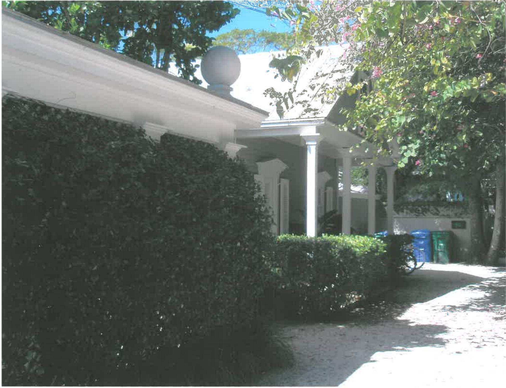
2 GECKO LANE Fence enclosing pool, original front facade
