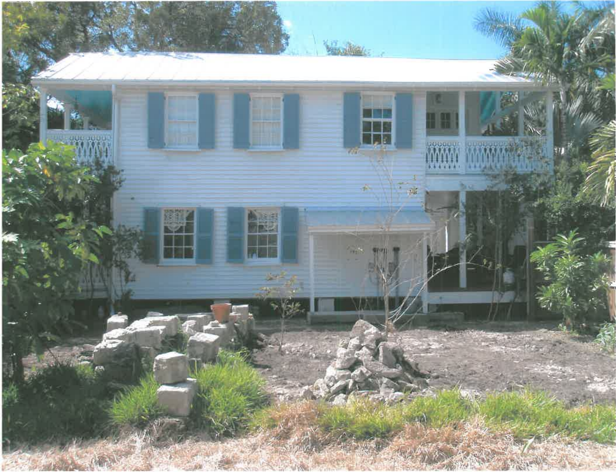
309 Caraballo Lane (Wrubbe Residence) NB side with lot in foreground 12
