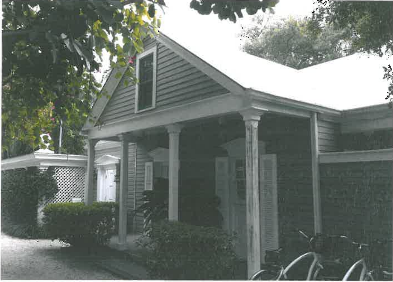
Original porch on front of Main House @ Gecko Lane.
