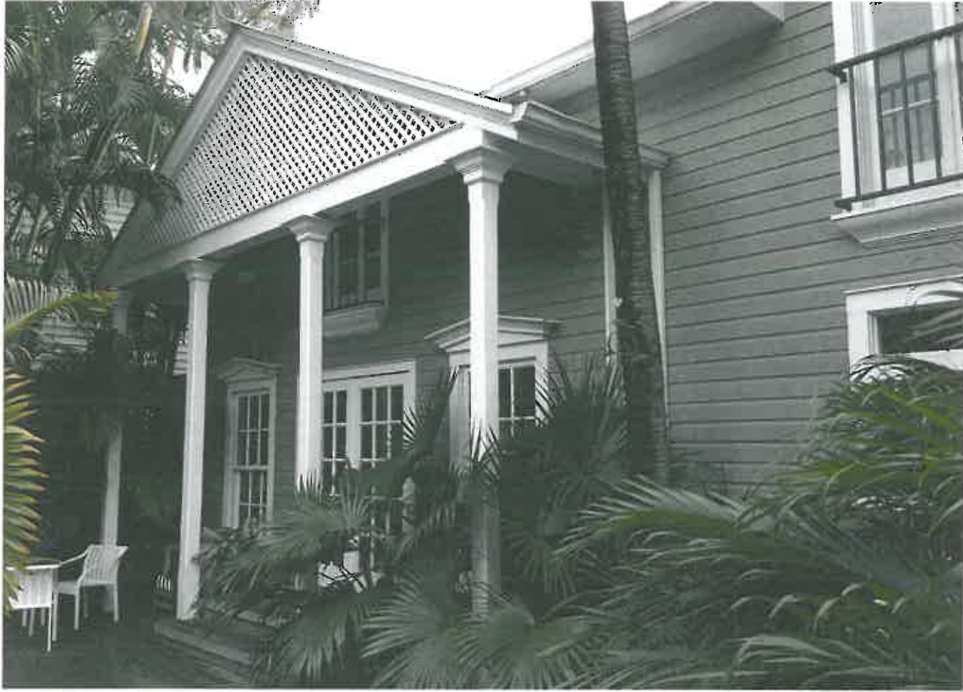
This is a porch addition to the Pool House, 1989. The new porch on the rear of Main House will be similar.
