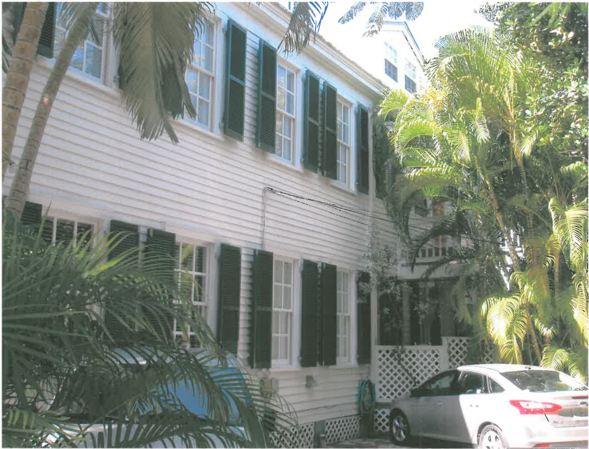
Side of 217 EATON ST along GECKO LANE
