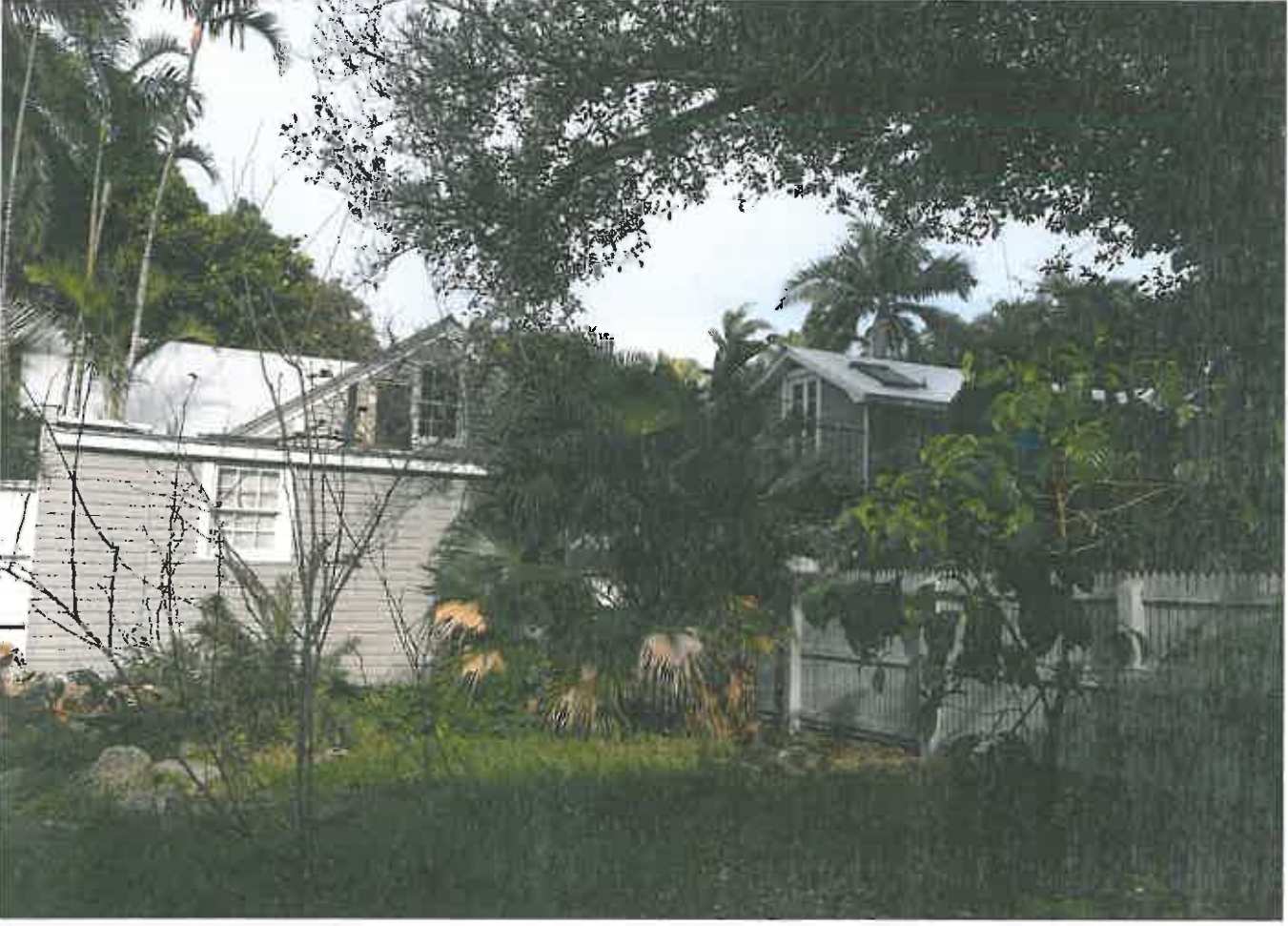
View of rear of original Main House from lot. One story addition to be removed.
