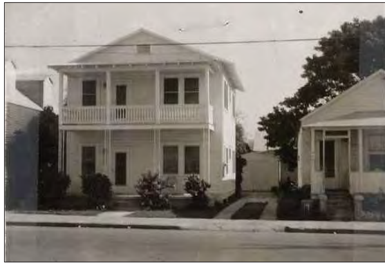
3 PHOTOGRAPH OF PREVIOUS HOUSE (C1965) A3 / SCALE: N.T.S.
