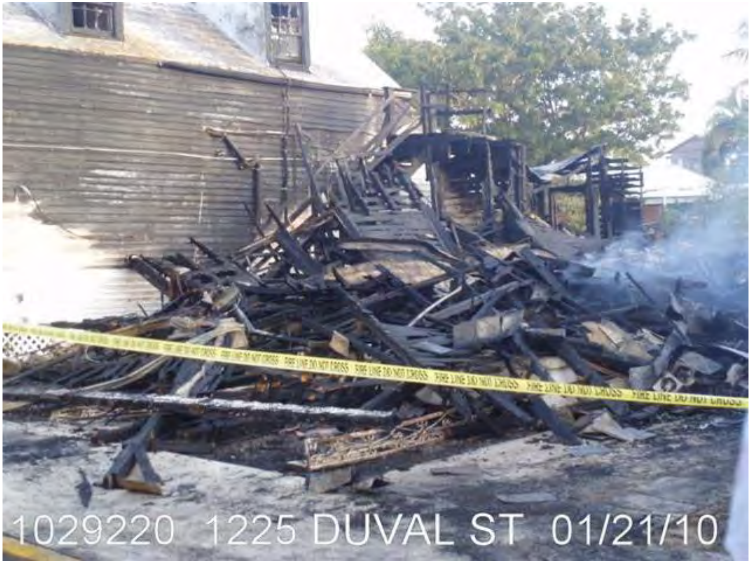
1225 Duval Street after a fire destroyed the historic house in January 2010.
