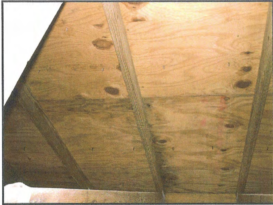
Photo No. 33 – Typical condition of roof deck and prefabricated wood trusses.
