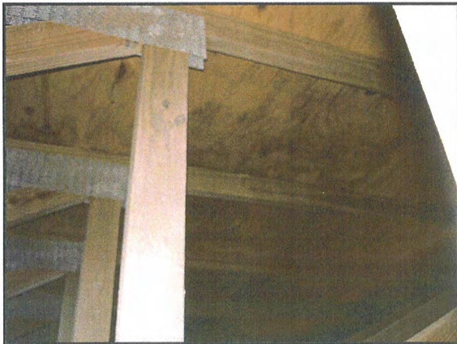
Photo No. 34 - Typical condition of roof deck and prefabricated wood trusses.
