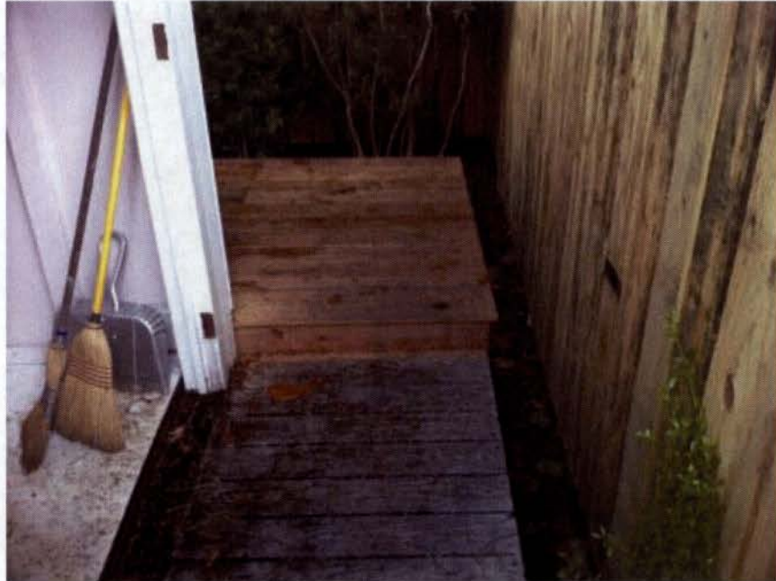
EXISTING DECK AT SHED TO REMAIN
