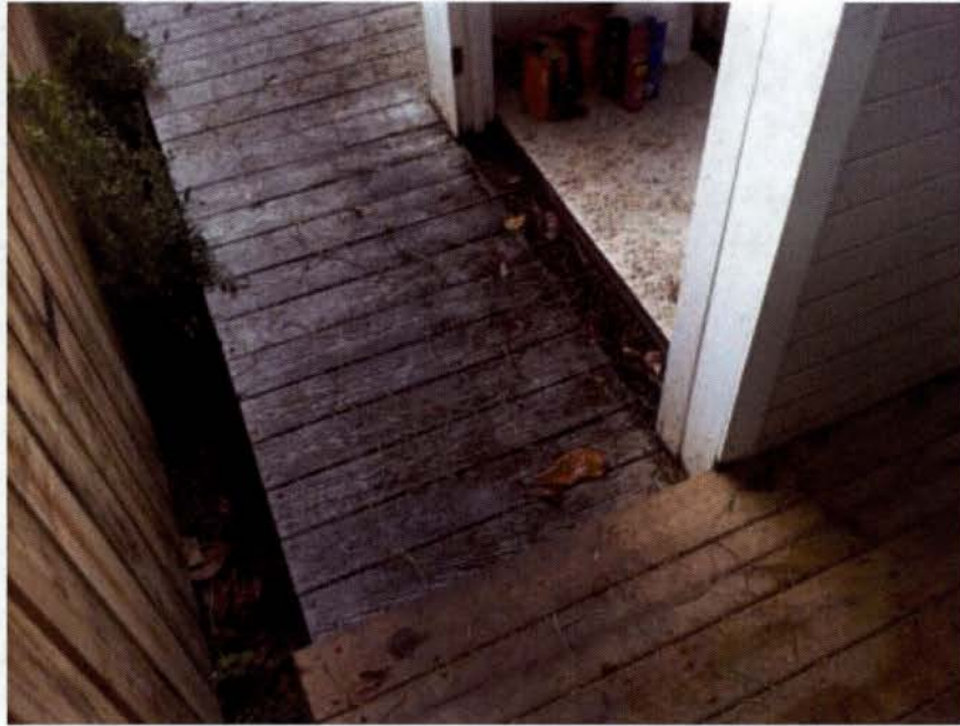
EXISTING DECK AT SHED TO REMAIN
