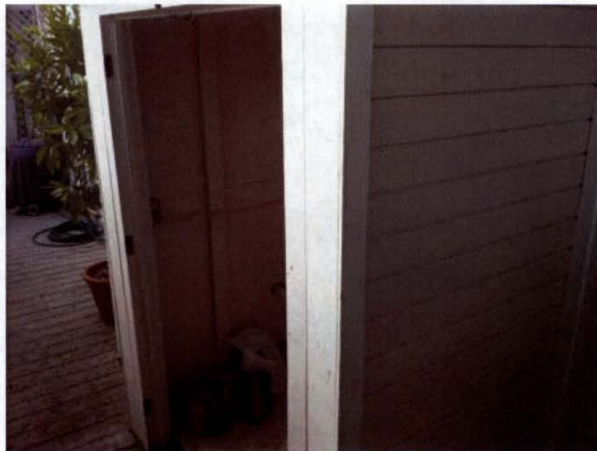
EXISTING DECK AT SHED TO REMAIN
