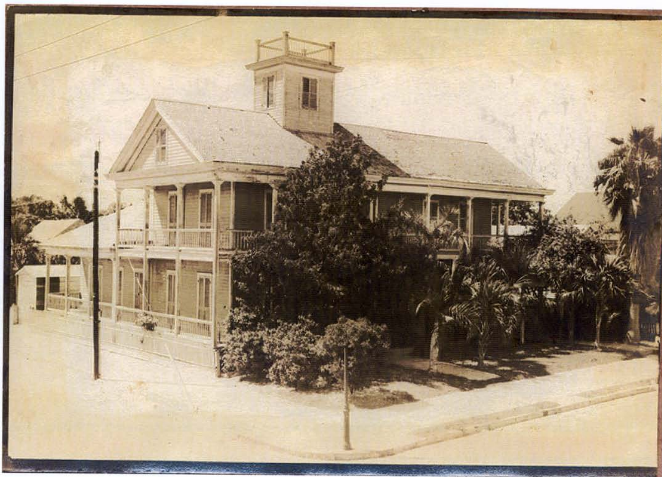
The Heritage House Collection, donated by the Campbell, Poirier and Pound families. The house at 730 Southard Street in the 1930s. From a collection of photographs taken or collected during the 1930s by the WPA workers in Key West.
