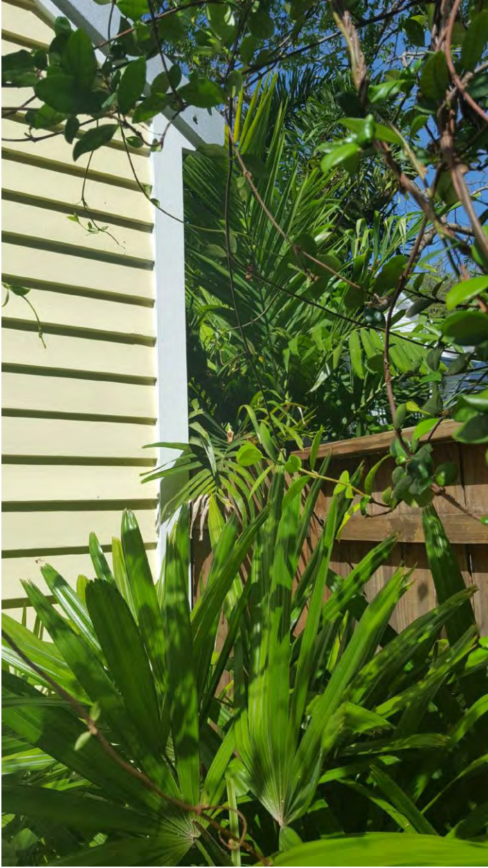
Existing structure on property line –North side
