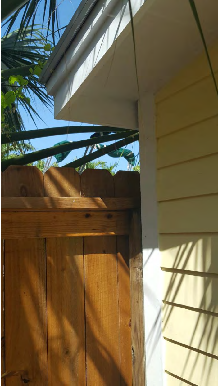
Existing structure on property line –West side
