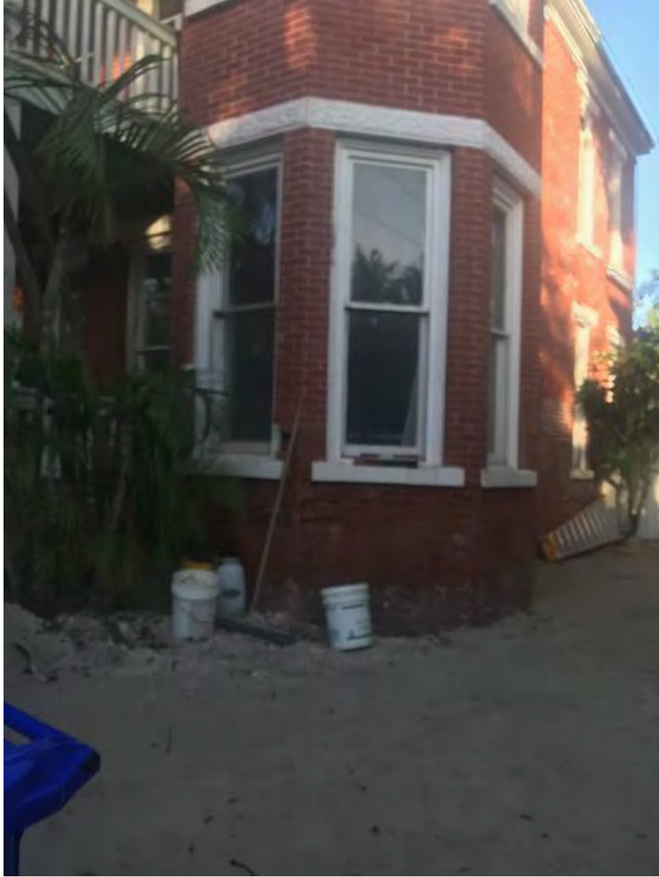
Current conditions front view of turret
