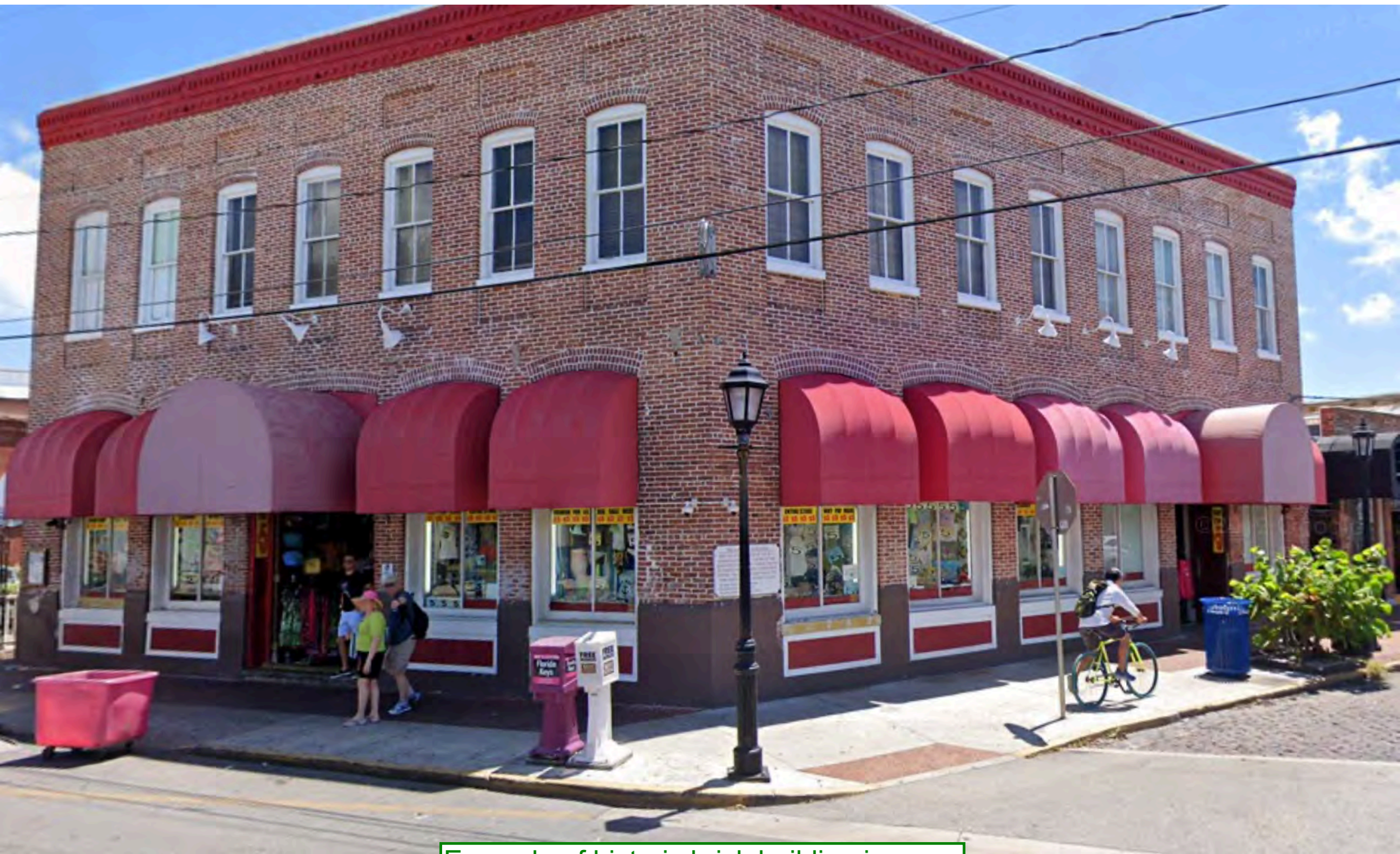
Example of historic brick building in historic Key West with similar stucco repair. 427 Front St.
