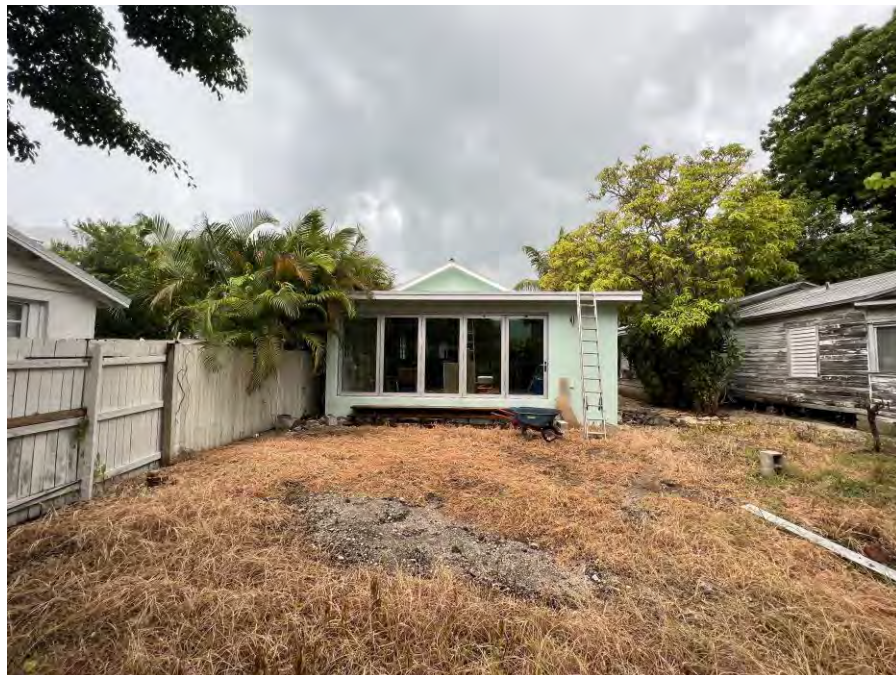
217 Eanes Lane – East Façade – Rear.
