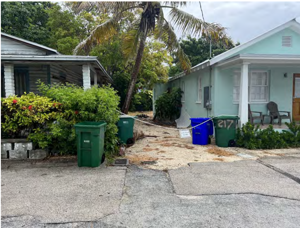
217 Eanes Lane – North Façade - Side.
