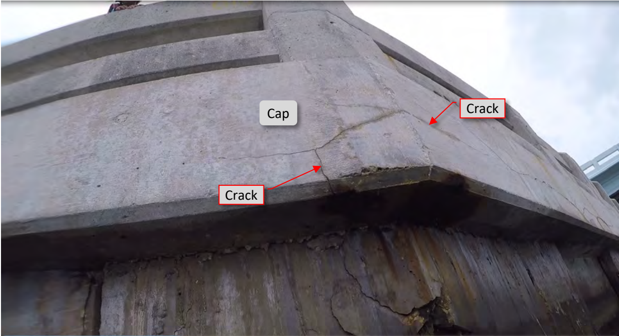
Figure 132: C11. STA 6+11. Crack at cap's vertical and bottom faces.
