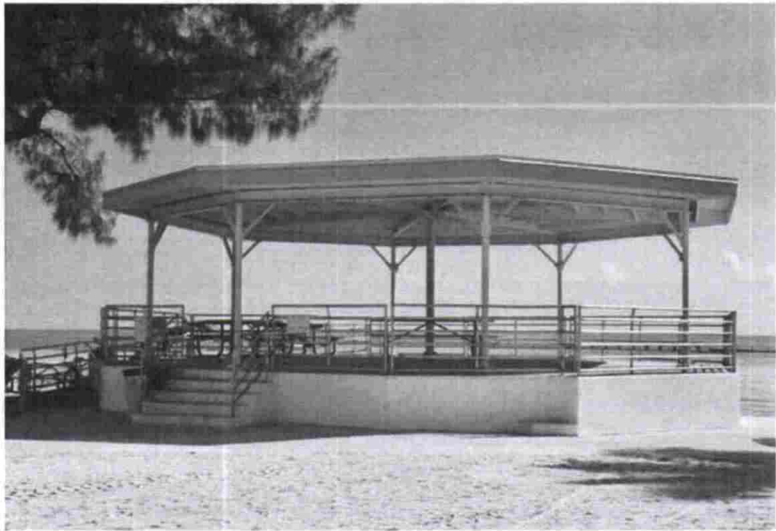
MO3430 east bandshell, view south, January 2017.
