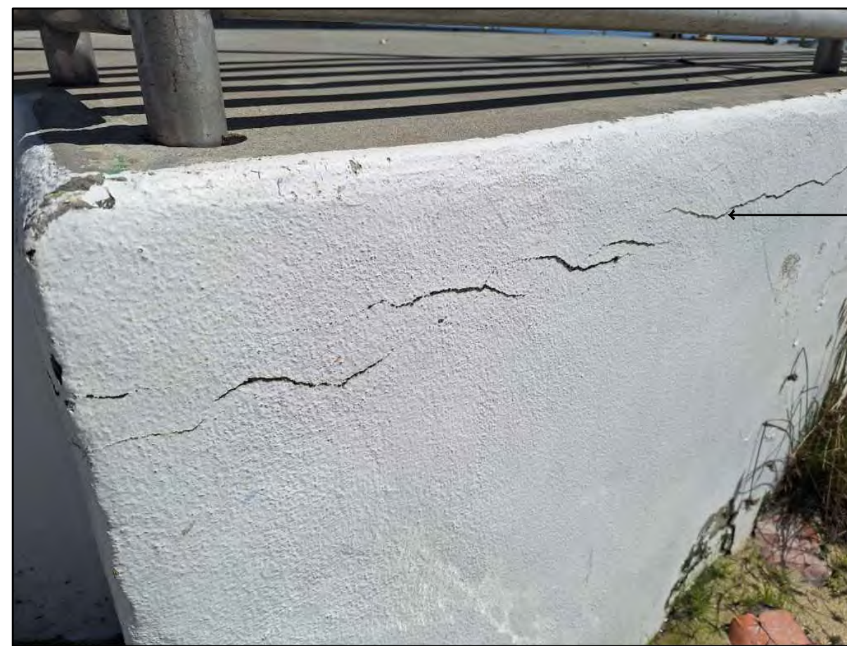
5 EAST PAVILION- DAMAGED STUCCO A5 SCALE: 1/4"=1'-0"
