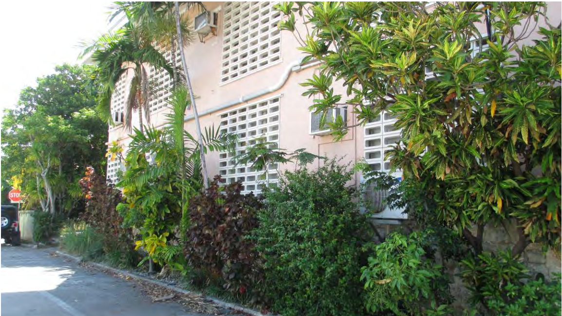
View of the north side of the existing building.
