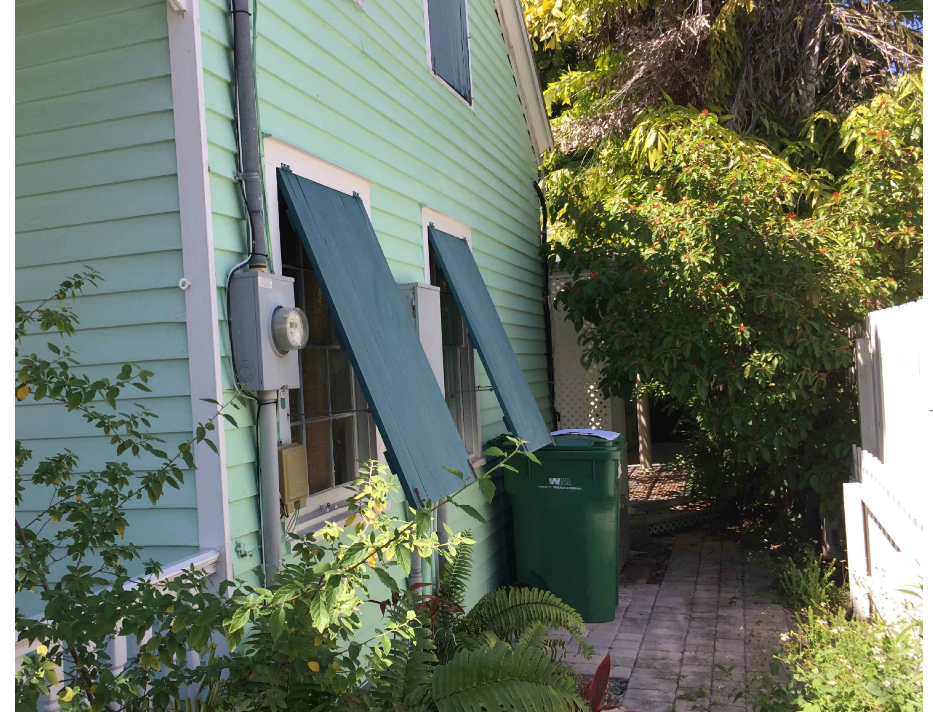
4 PHOTOGRAPH OF EXISTING EAST ELEVATION
