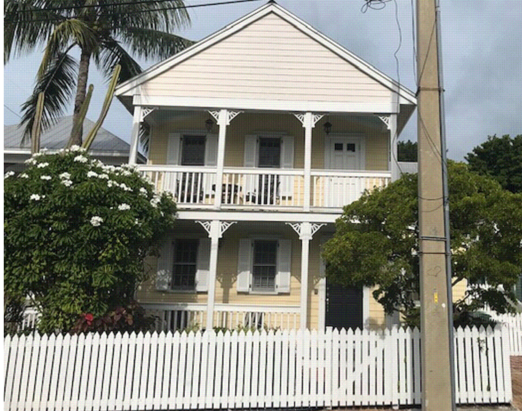
5 PHOTOGRAPH OF ADJACENT PROPERTY TO THE WEST
