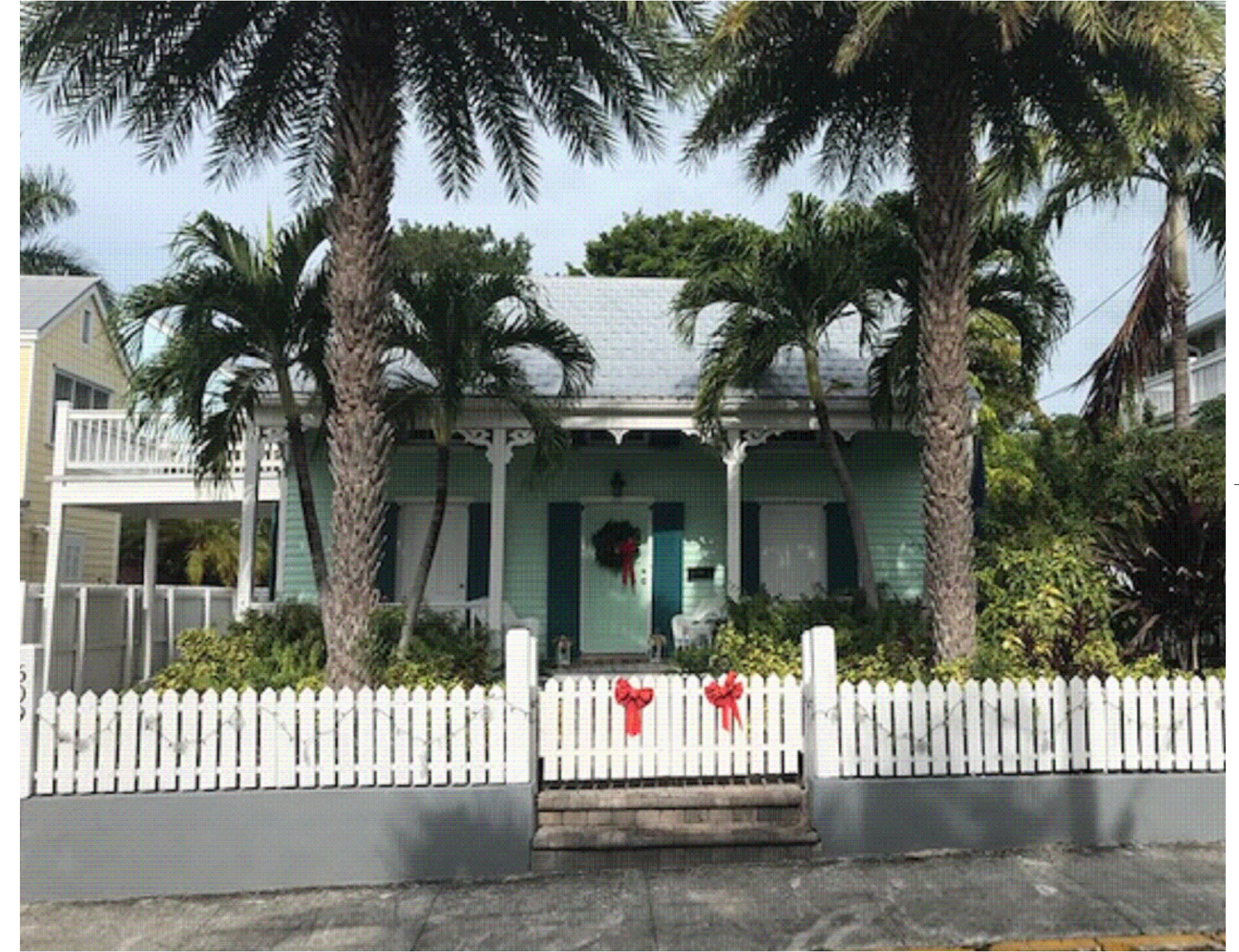
1 PHOTOGRAPH OF EXISTING ANGELA STREET ELEVATION
