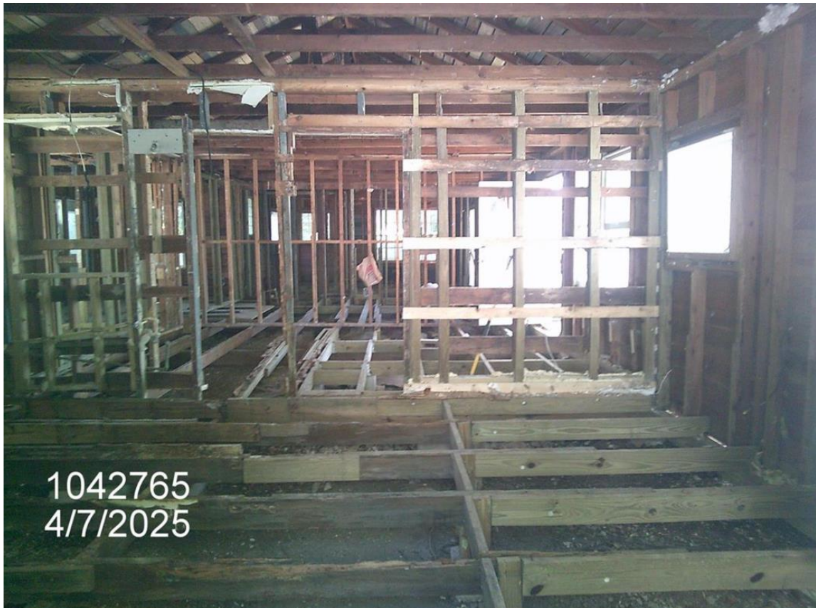
Photo of property already demolished. Property Appraisers website 04/07/25.
