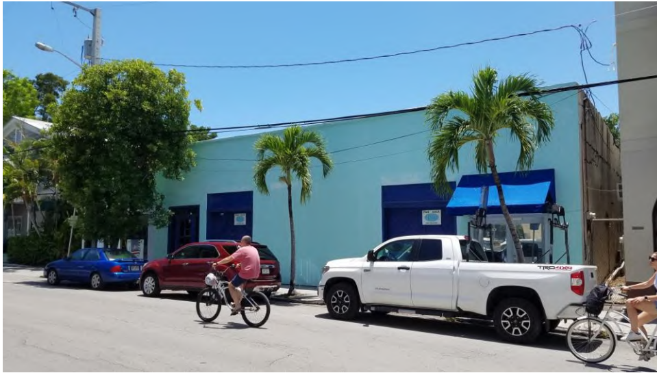
Simonton Street façade.
