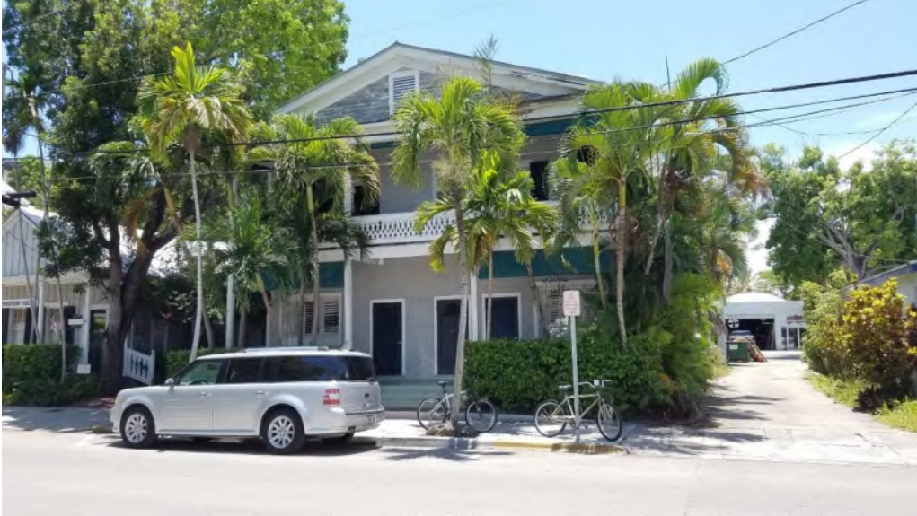
Adjacent building, 320 Simonton.
