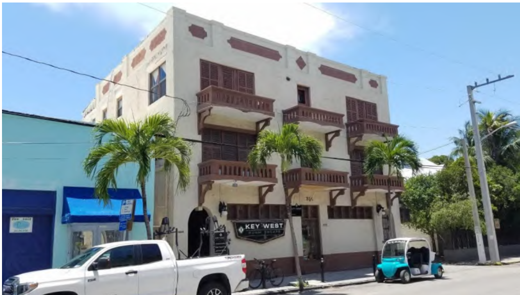
Adjacent building, 314 Simonton
