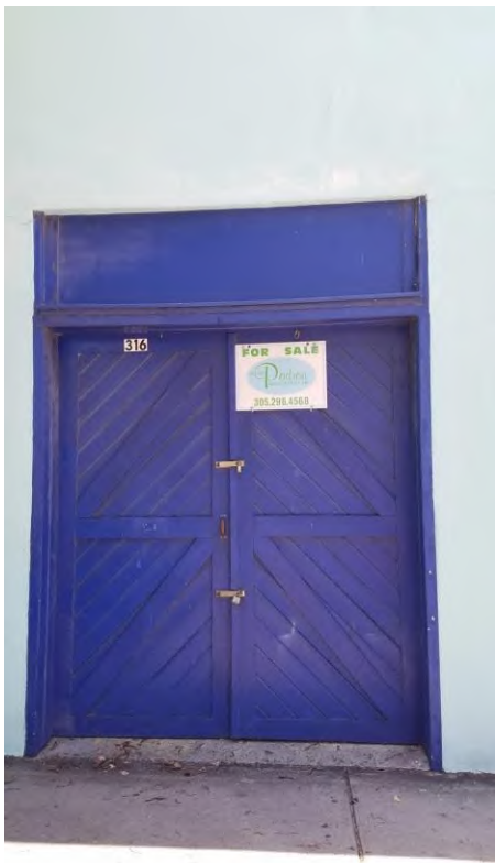
Building 1 Historic Warehouse Door
