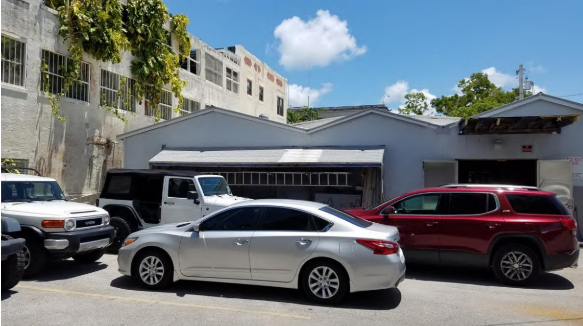
Building 3 Exterior, east side
