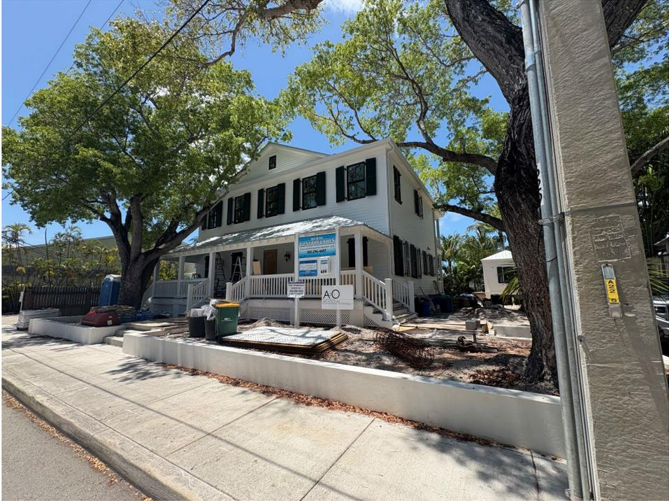
629 DEY ST | METAL FENCE TO BE INSTALLED ON CONCRETE KNEE WALL AT FRONT PROPERTY LINE.
