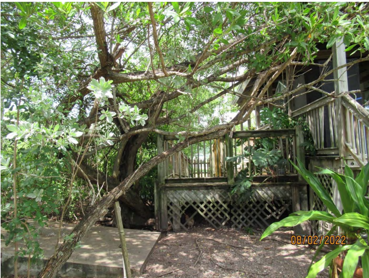
Photo looking west at the south side of the existing structure, area will need to be properly trimmed prior to construction and demo work.
