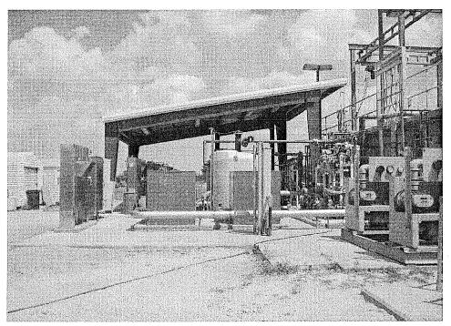
The Glades County Waste Water Treatment Plant included the installation of Membrane Bioreactor System (MBR) into the existing aeration train. The installation provided a 135,000 GPD expansion to the existing facility.
