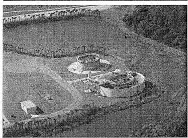
The Ave Maria Water Treatment Plant project included the construction of a water treatment facility for Ave Maria University and the surrounding community. Construction included an operations building, electrical building, chemical storage building, degasification foundations, package plant slabs, filter structures, a chlorine basin, high service pump slabs, and water well slabs. Several of the above structures required deep excavation for the foundations.
