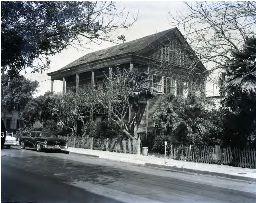
1960's 610 Caroline Street – No carport/ Garage
