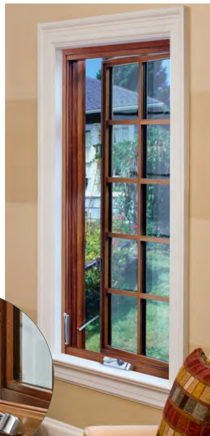
INTERIOR VIEW. WOCD LIMITS THE SASH OPENING TO LESS THAN 4 INCHES
