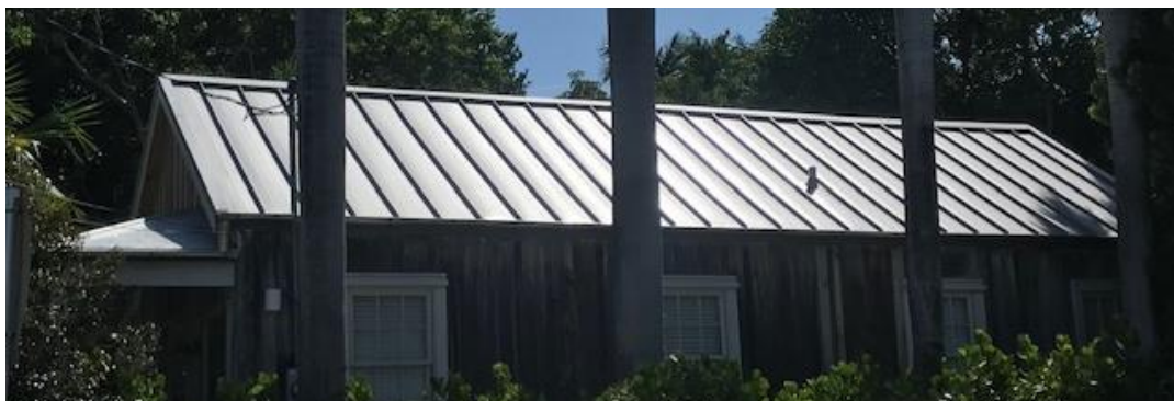
1400 Virginia Street after with standing seam.
