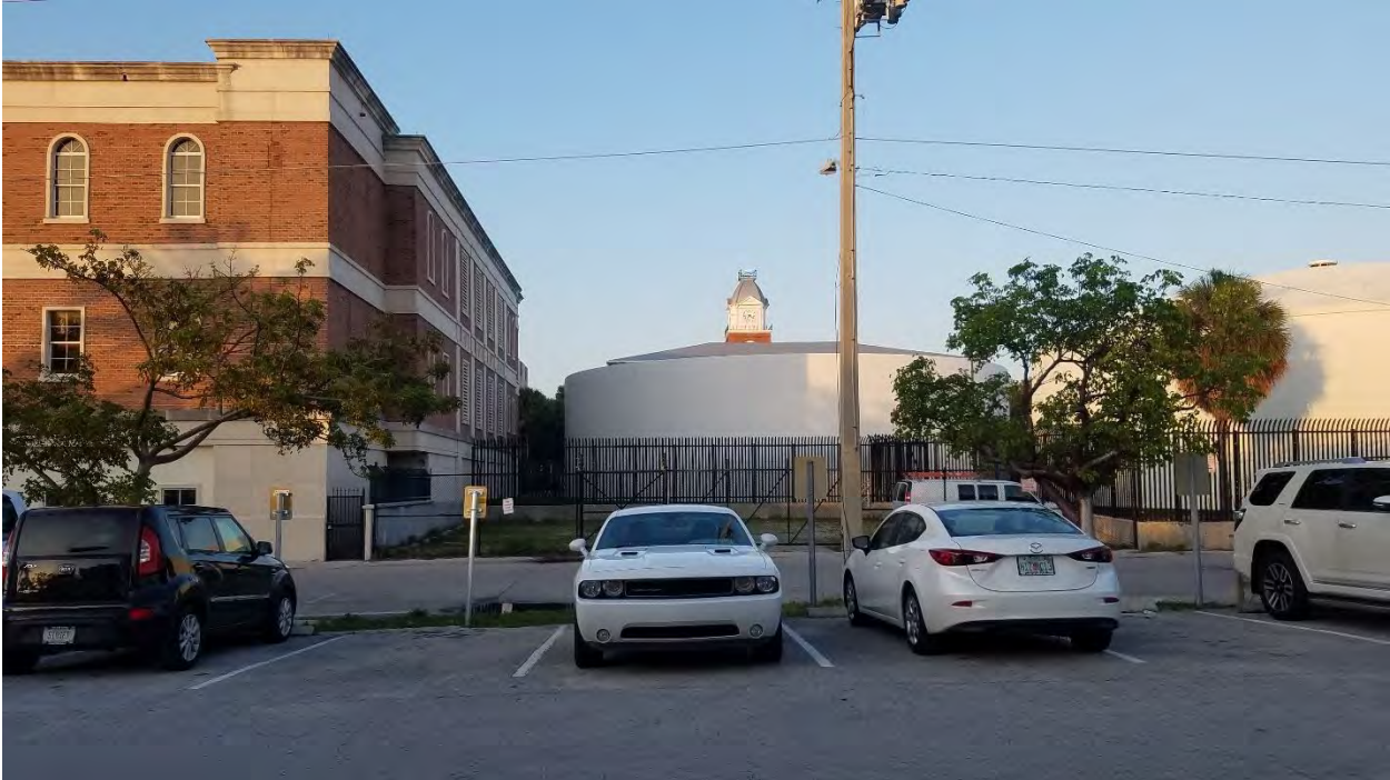
Adjacent building: A large FKAA water tank is located to the right of the site, as well as behind the site.
