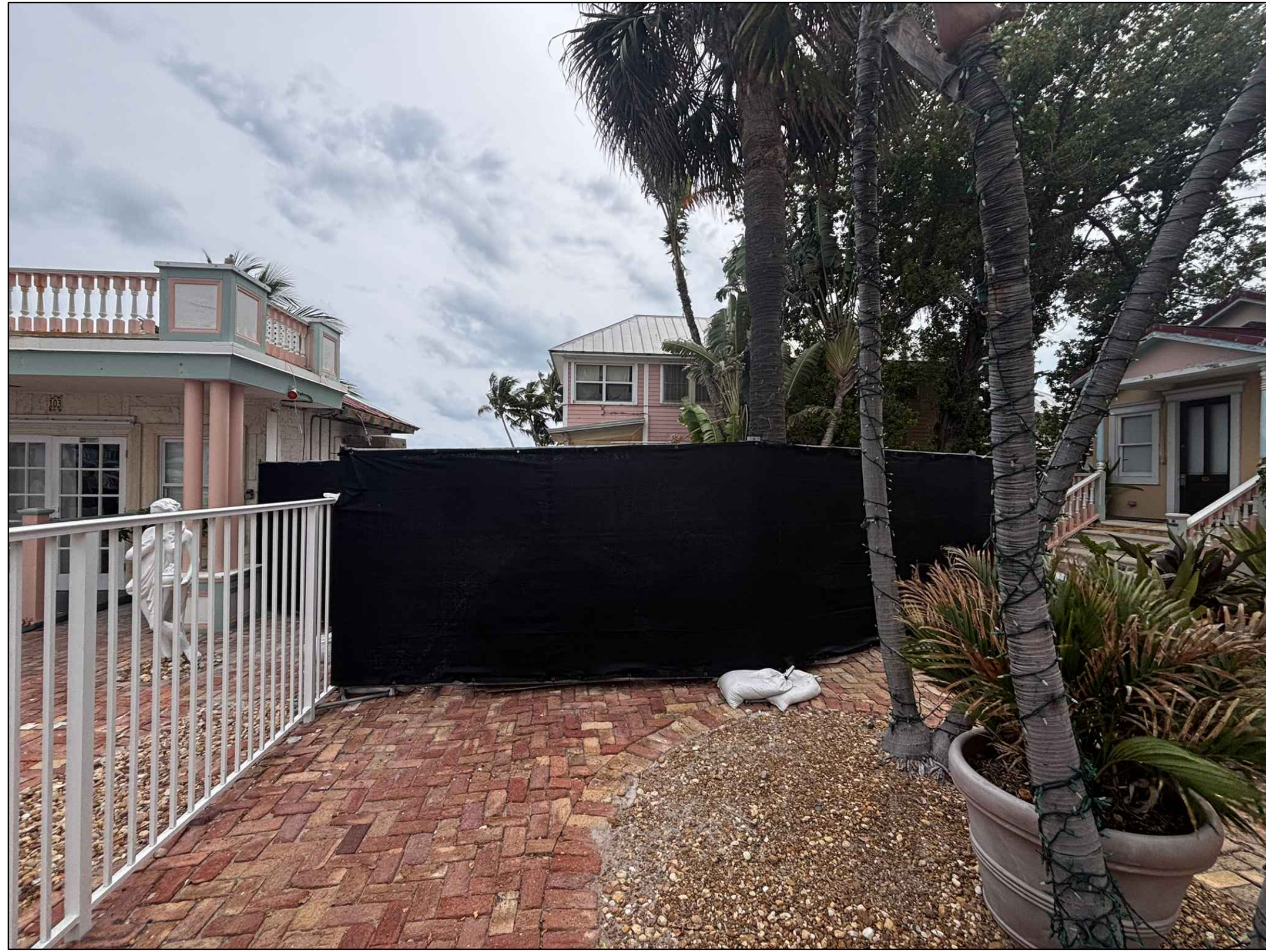
3 VIEW FROM EAST SIDE OF THE PROPERTY A4 SCALE: 1/4"=1'-0"
