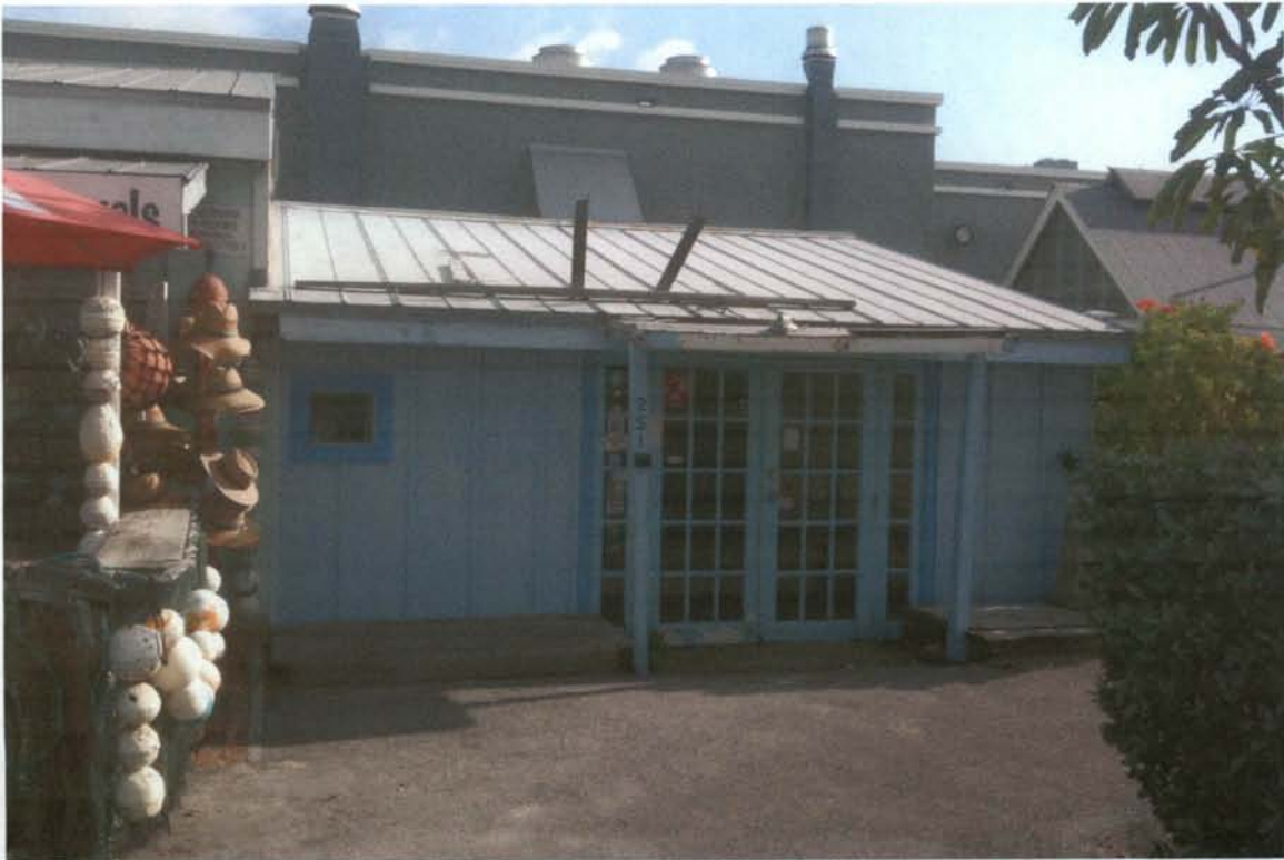
BUILDING TO BE DEMOLISHED
