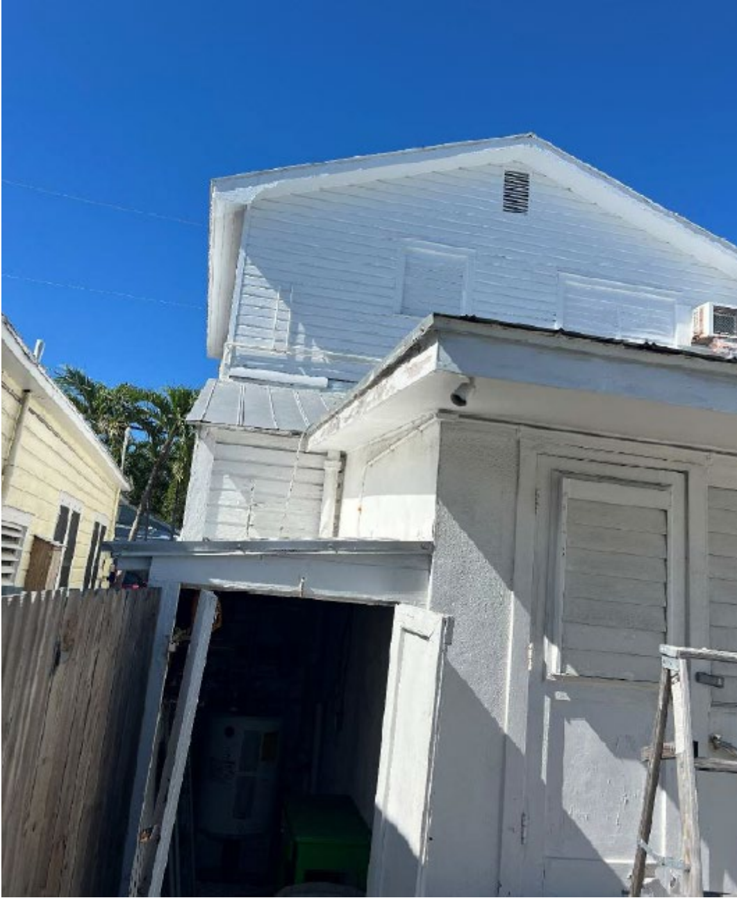
Phot of Rear of Property Under Review Showing both Rear Rooflines.
