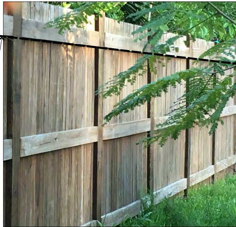
PHOTO DETAIL 1- 616 EATON STREET SIDE
