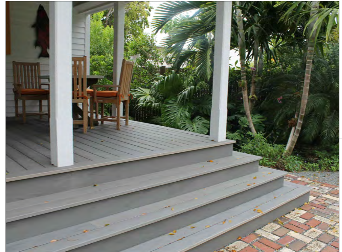
PHOTO DETAIL 3- FROM POOL HOUSE DECK
