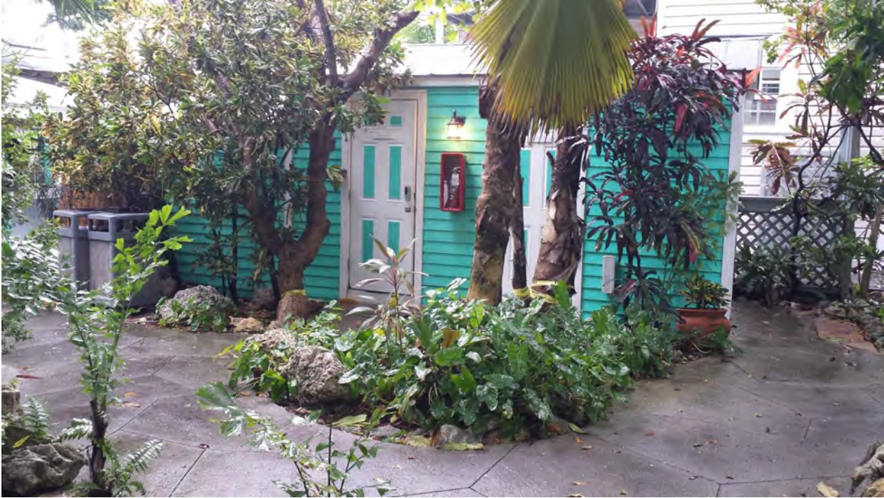
EXISTING STRUCTURE - FRONT VIEW
