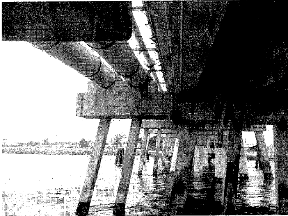
The City of Key West Sewer Bridge is the two pilings and concrete support for the two pipes on the left of the picture. It sits immediately adjacent to the Navy's roadway bridge to Fleming Key
