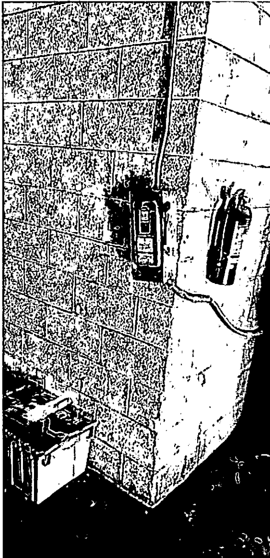
Figure 39. Example of the damaged disconnect enclosure and conduit (in the way of forklift traffic) needs to be moved, replaced or abandoned. The equipment connected may not be in service.
