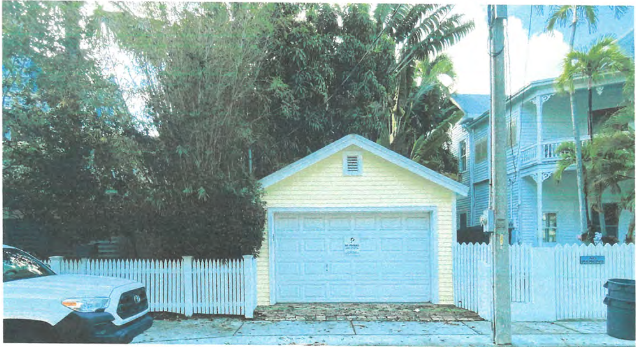
620 Dey Street - Garage
