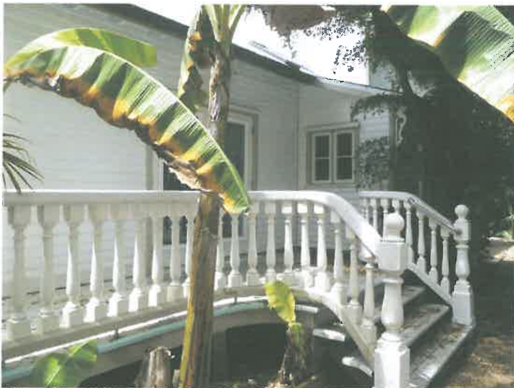
Non-Historic Side Porch (To be replaced)
