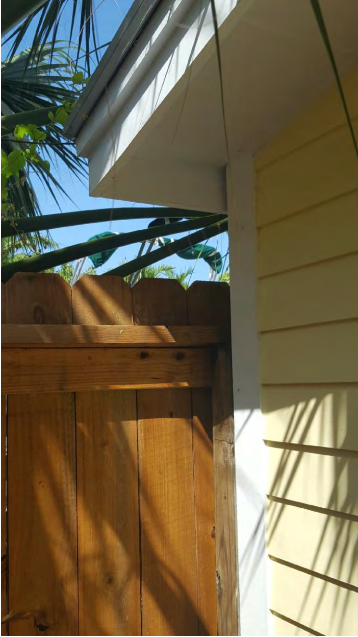
Existing structure on property line –West side
