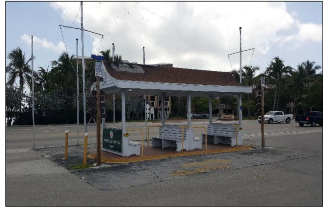
Images of the trolley station shelter, flag poles, and billboard sign to remain.
