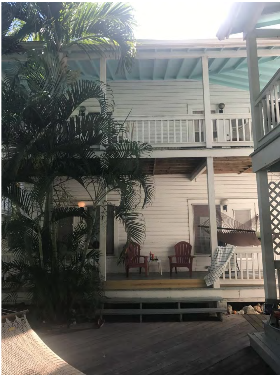
1218 Duval Street REAR VIEW
