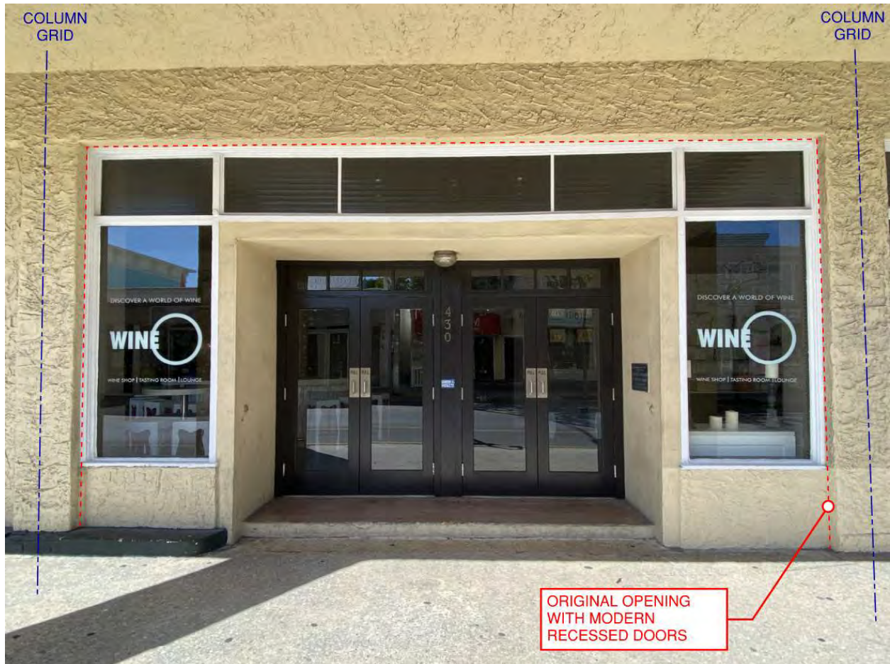
Bay 6 – existing conditions
