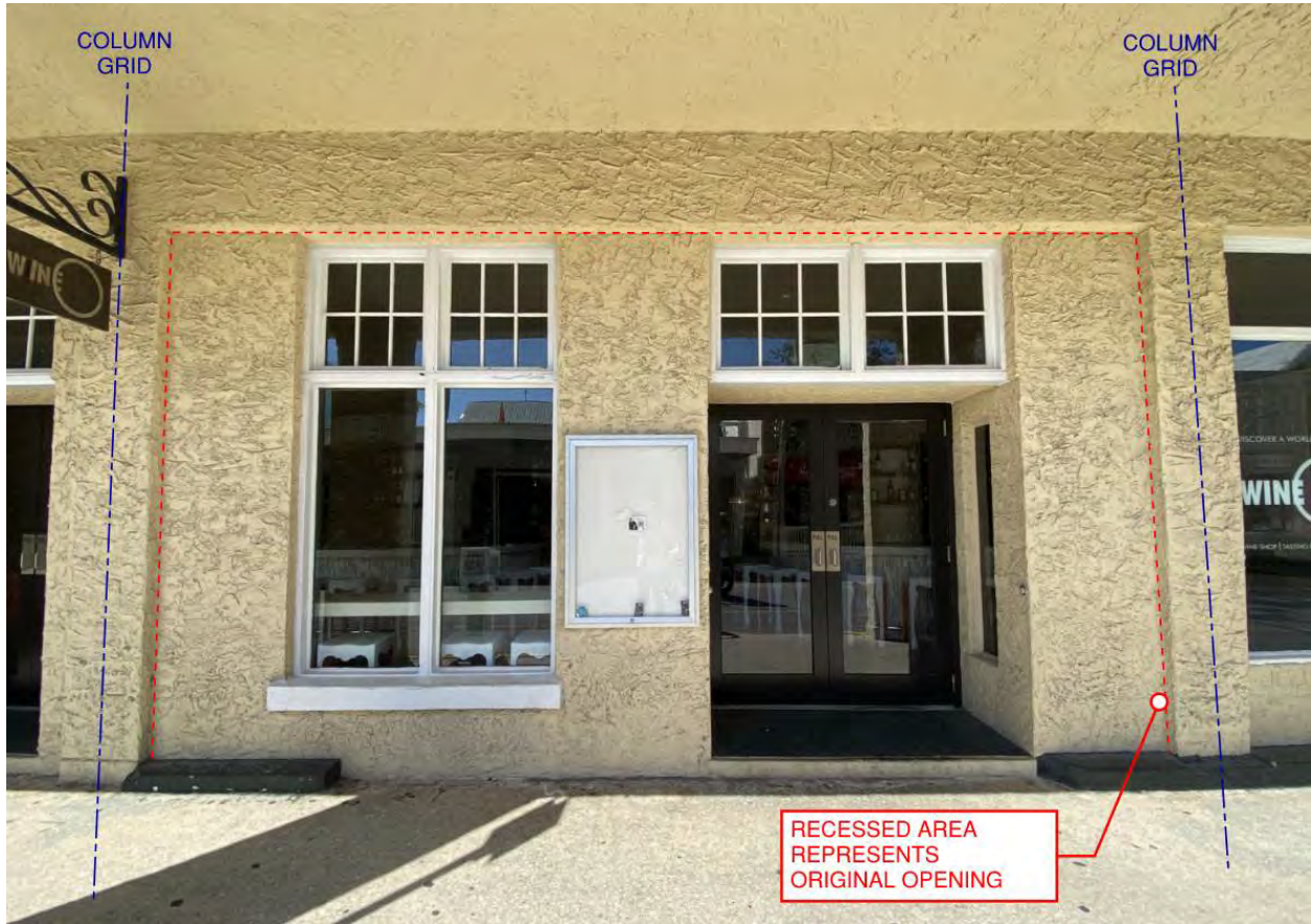
Bay 5 – existing conditions
