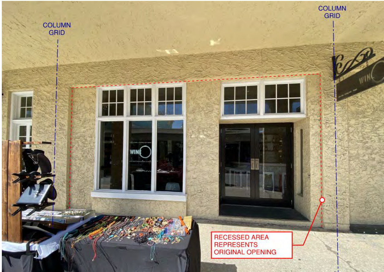
Bay 4 – existing conditions
