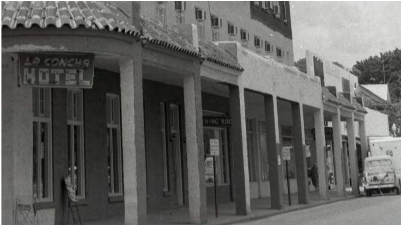
Detail of 1957 photograph. Monroe County Library.
