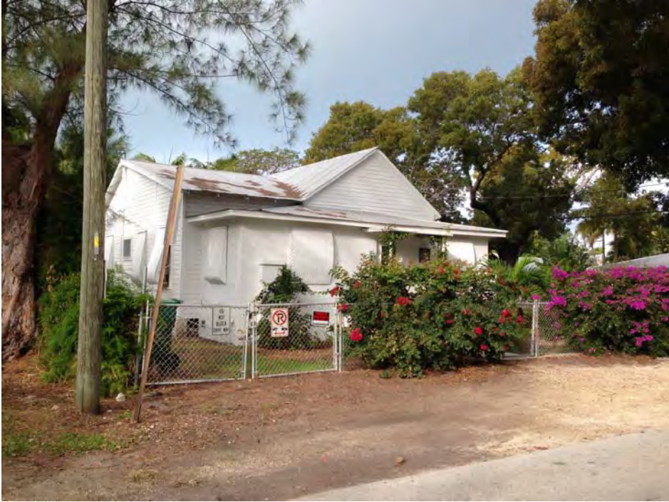
View of adjacent property to the north (right side)
