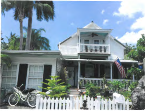
Front View of 1212 Georgia Street. Deck is not visible from street level. New Walkway can be seen to the left of existing Center Porch. A corresponding Walkway is planned for right of Center Porch for aesthetic balance
