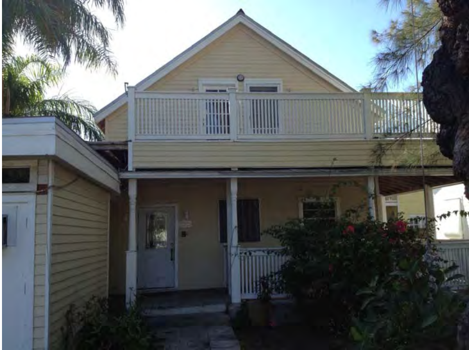
Current street side view of the structure
