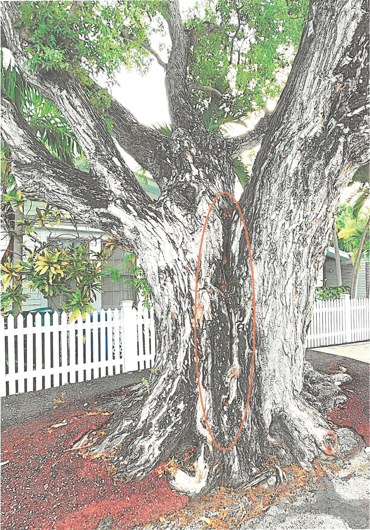
Photo 4. View of the vertical crack in the trunk as viewed from Frances Street.
