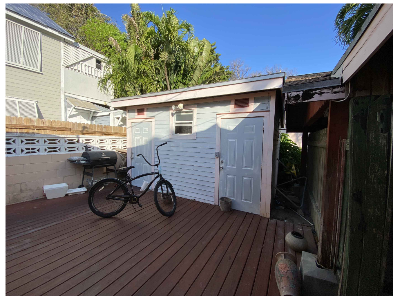
4 EXISTING ACCESSORY STRUCTURE
