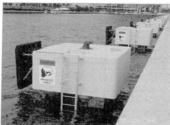
Bicentennial Park Large Vessel Mooring Facility
