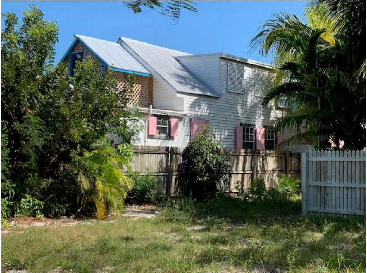
Looking at front right corner from center – view of 910 Thomas Street.
