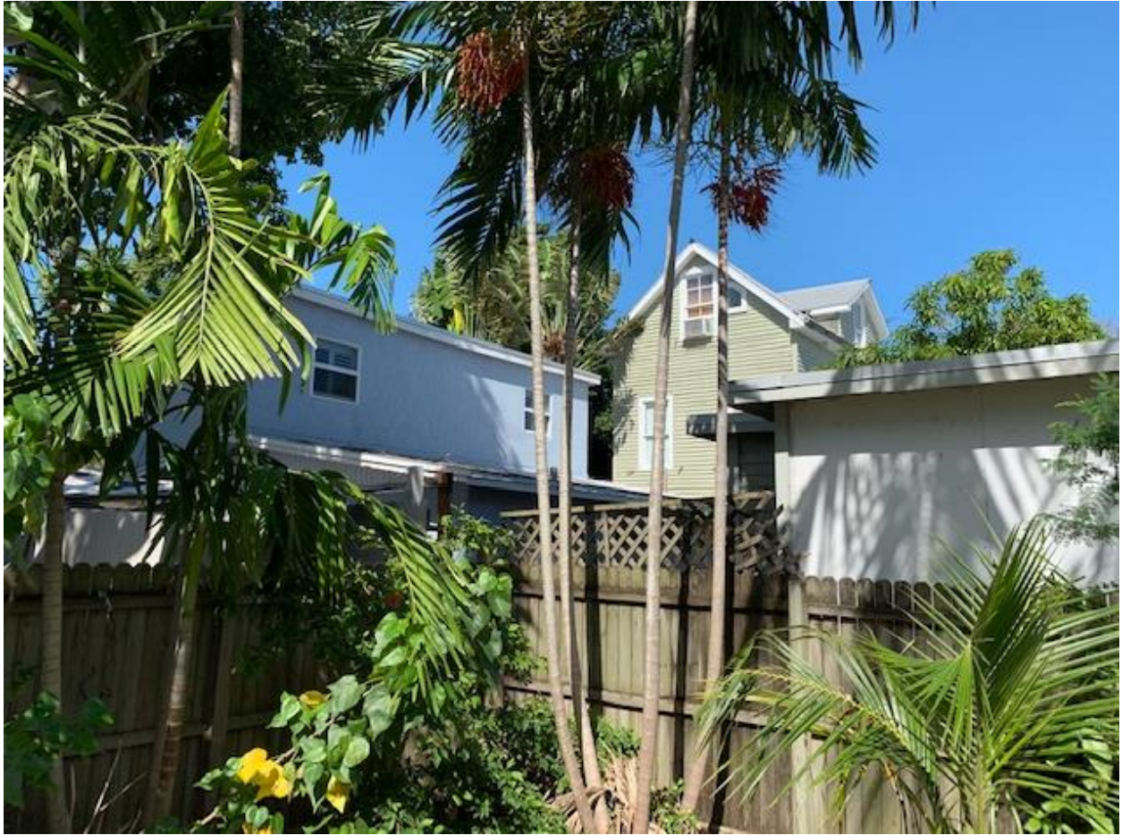
Back right corner – view of 3 Hutchinson Lane and 219 Olivia Street.
