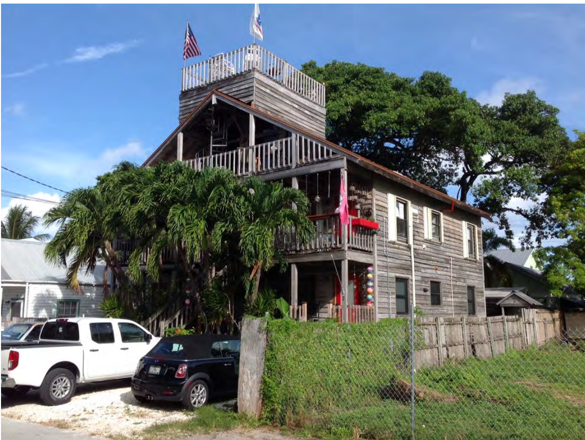
313 CATHERINE STREET (NEIGHBOR TO WEST) – 2 ½ STORY MULTI UNIT RESIDENTIAL
