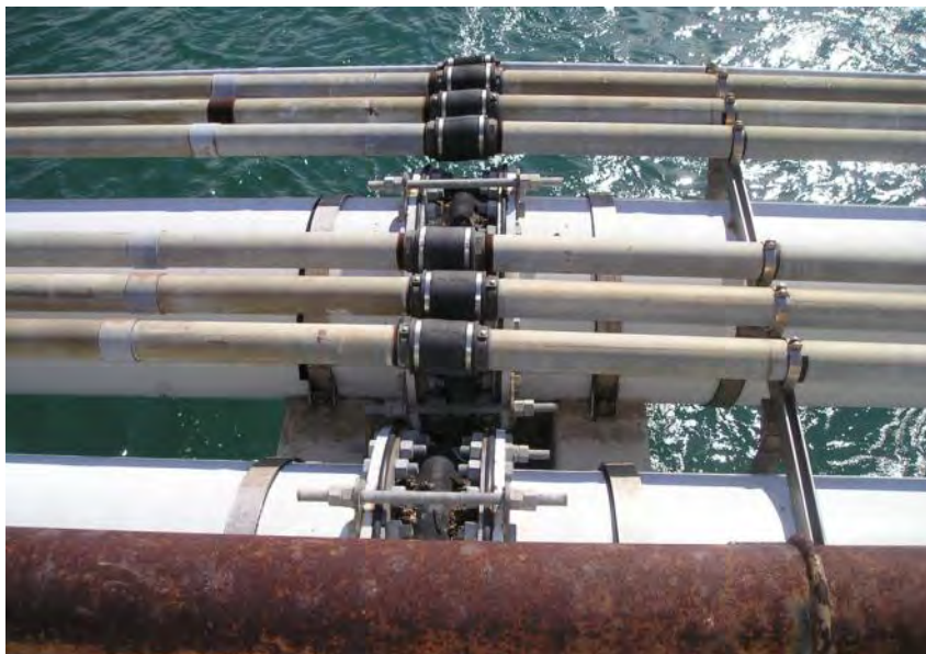
Photo No. 42: Top view of Pile Cap 8-9.
