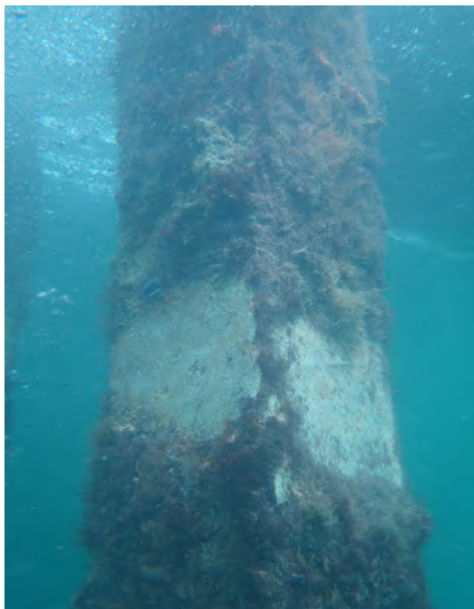
Photo No. 28: View of Southeast Corner of Pile 10.
