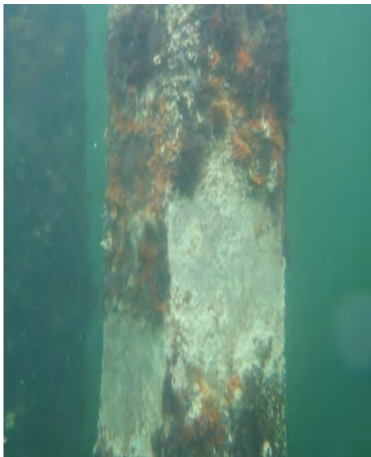
Photo No. 8: East Face of Pile 4, upper portion of marine growth removed.
