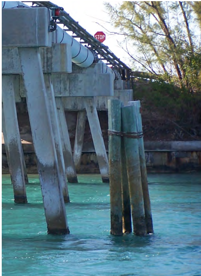
Photo No. 48: Existing Timber Pile Dolphin Fender
