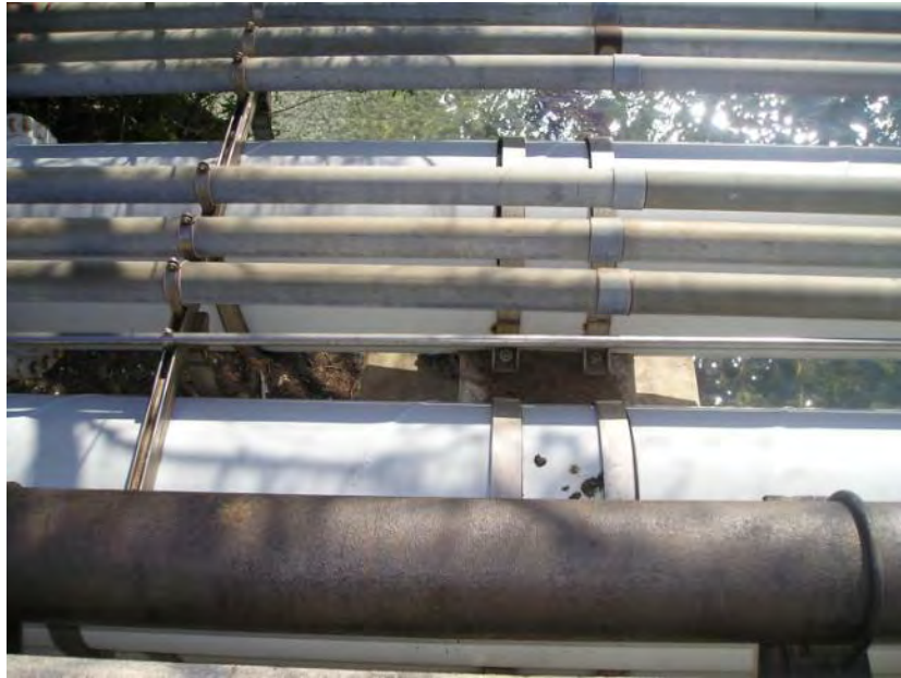
Photo No. 33: Top View of Pile Cap 12-13, showing the two 30-in water mains and numerous electrical conduit.
