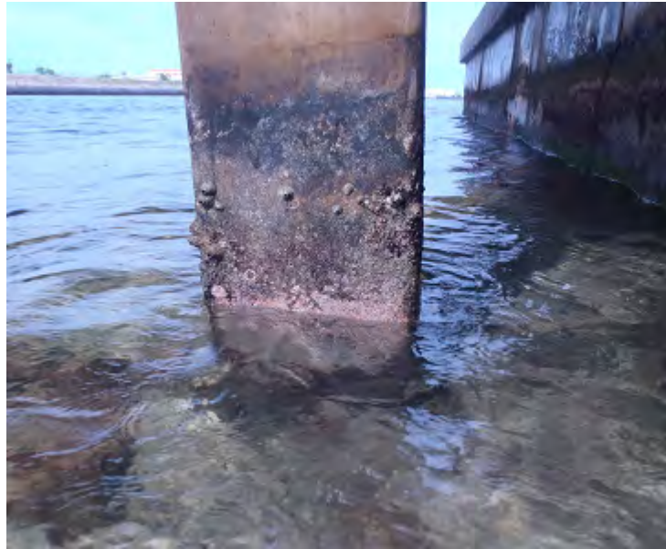
Photo No. 2: East Face of Pile 13.
