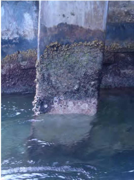
Photo No. 30: View of Pile 14 North Face above water.
