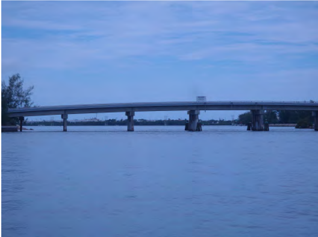
Photo No. 1: Fleming Key Bridge taken from the West Side.
