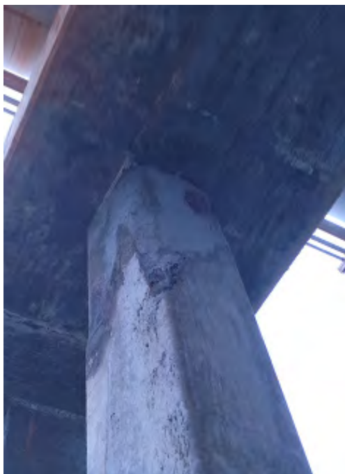
Photo No. 18: Northwest Corner of Pile 6, where the top of the pile intersects the concrete pile cap.
