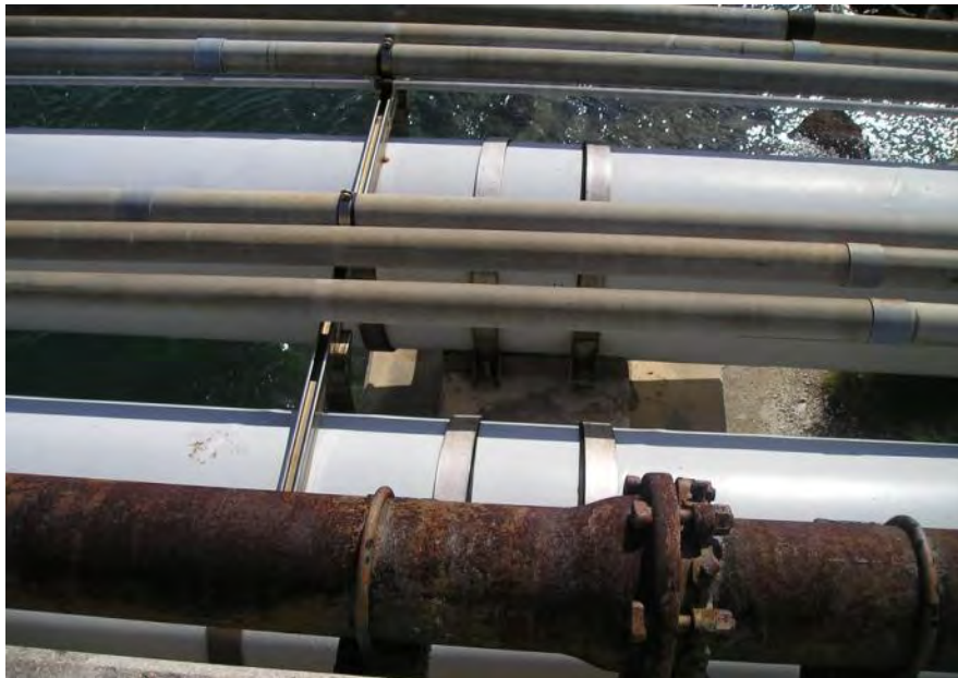
Photo No. 45: Top view of Pile Cap 14-15.
