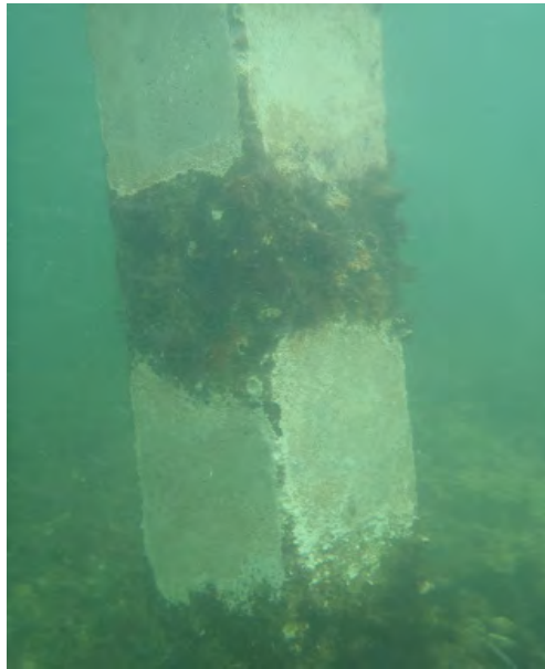
Photo No. 6: South Face of Pile 1, with two 12 inch bands of marine growth removed.
