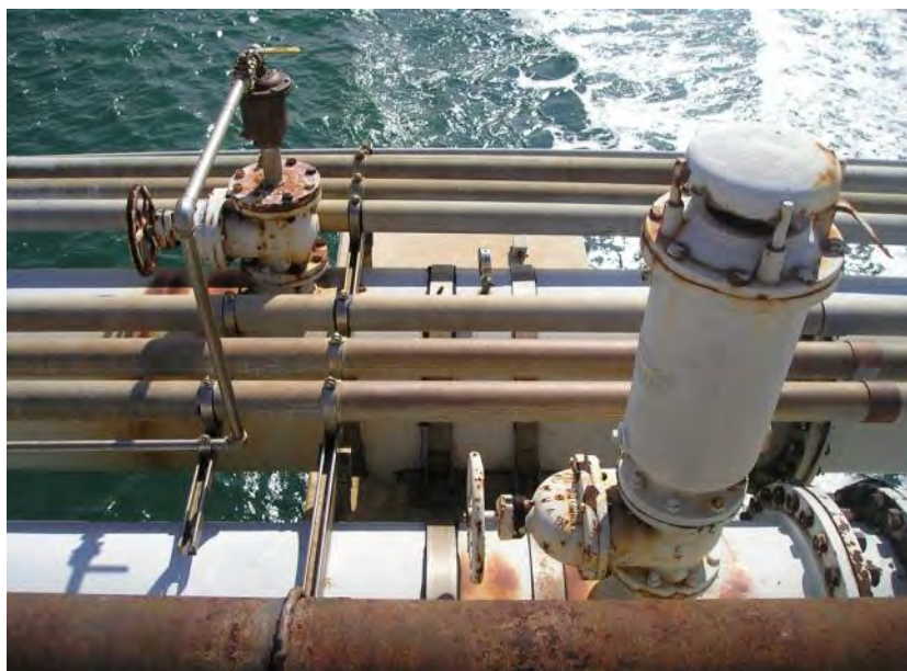
Photo No. 39: Top view of Pile Cap 5-6-7.
