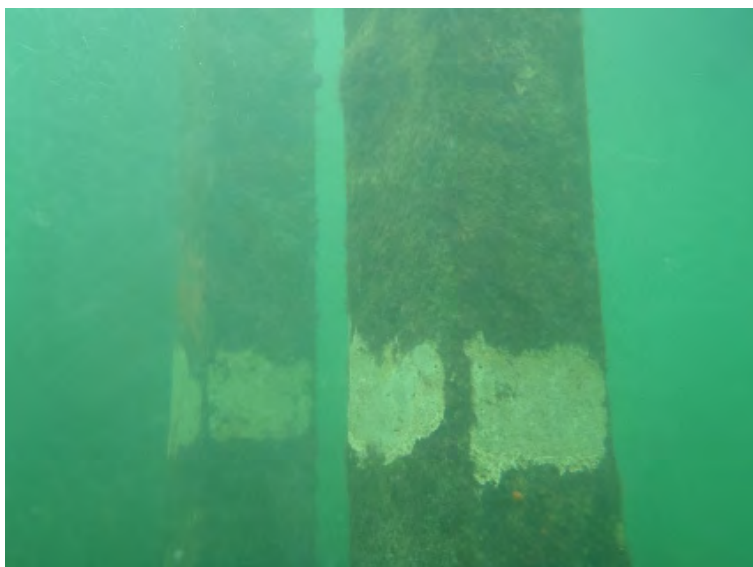
Photo No. 12: Southeast Corner of Pile 6, with no visible damage.
