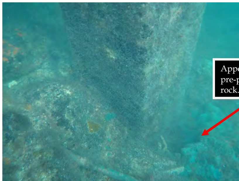
Photo No. 32: Typical bottom conditions at precast concrete pile, before cleaning. The bottom or mudline consists of rock, most likely coral or limestone; and it appears the rock was pre-punched before driving the pile.
