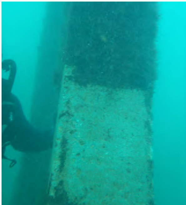
Photo No. 24: View of East Face of Pile 9.
