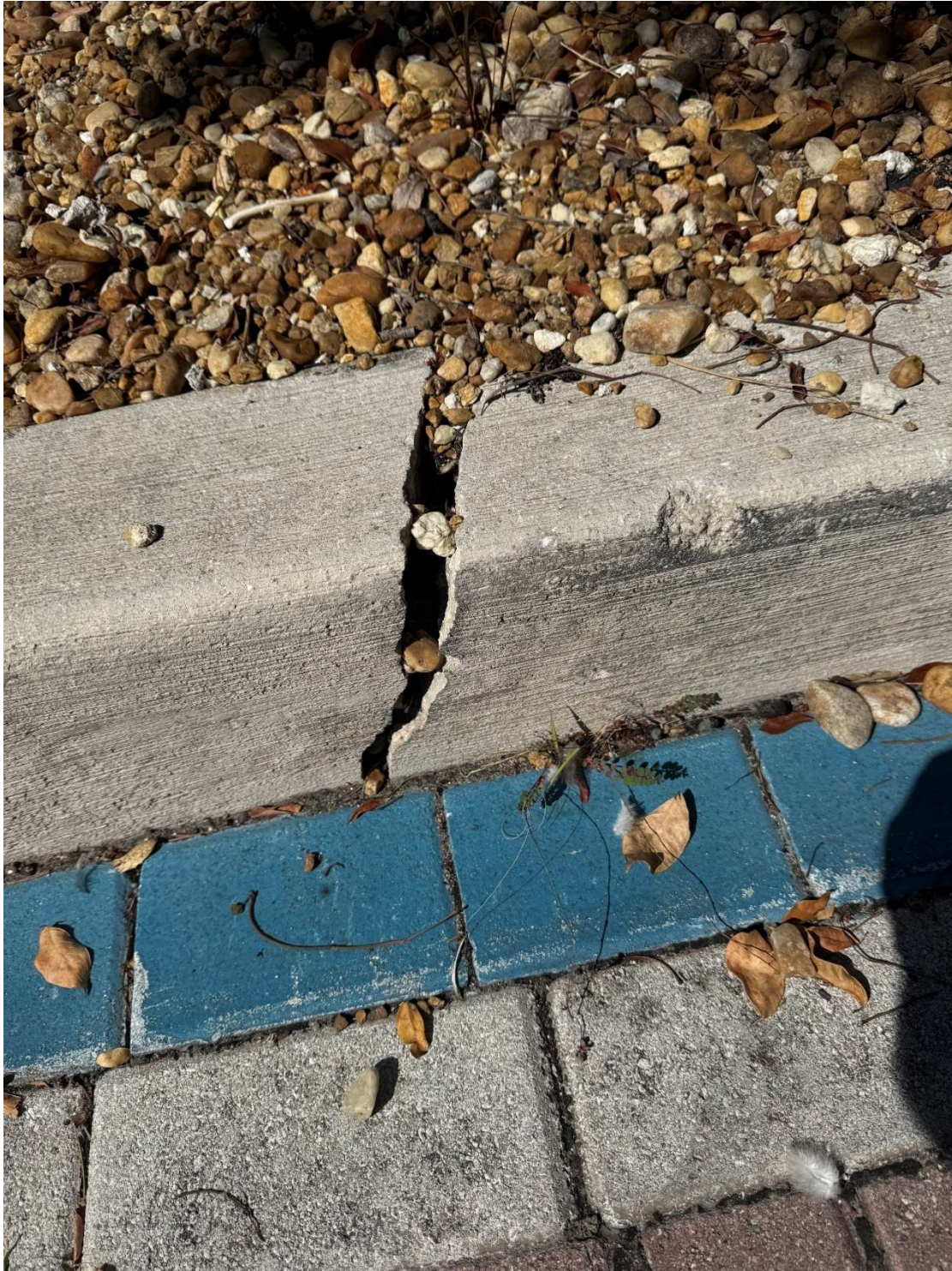
Roots that want to grow so badly, they can crack concrete. Gumbo Limbo #2
