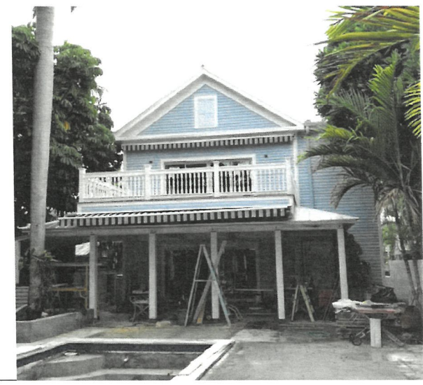
626 WILLIAMS STREET, REAR ELEVATION
