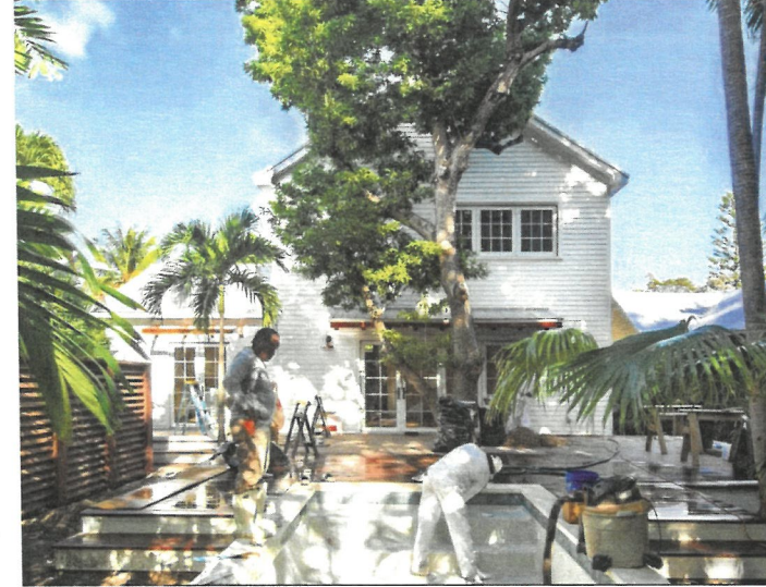
618 WILLIAMS STREET, REAR ELEVATION
