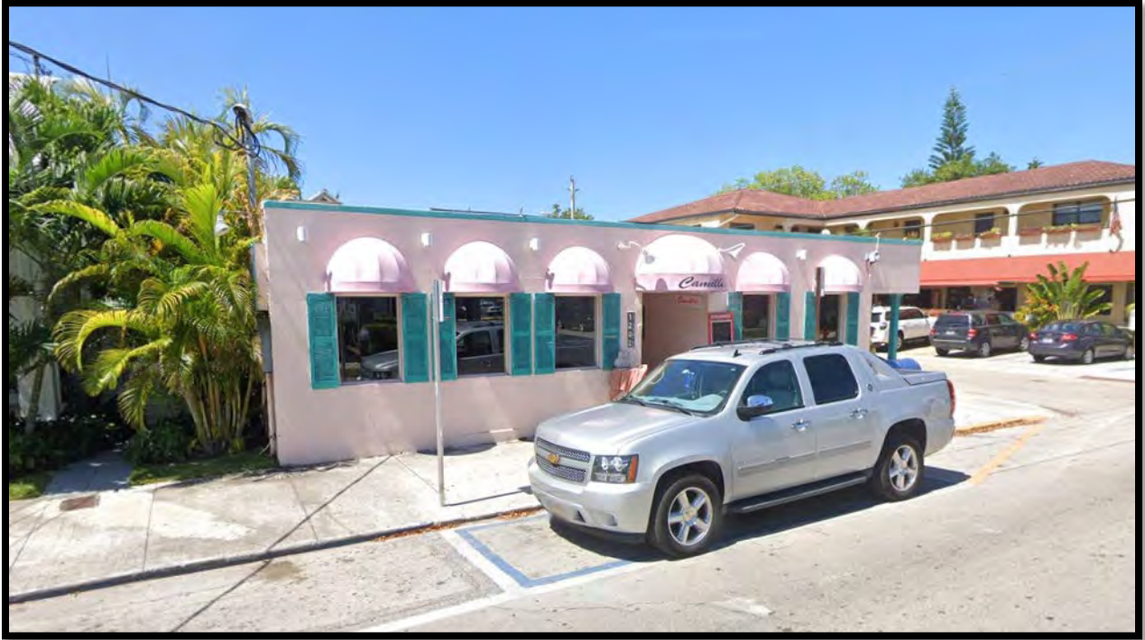
Front (Northeast) Elevation
