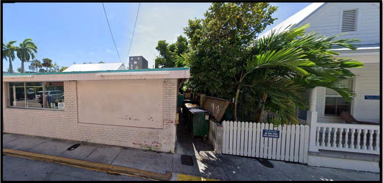
Streetside (Catherine) & Rear (Southwest) Elevation
