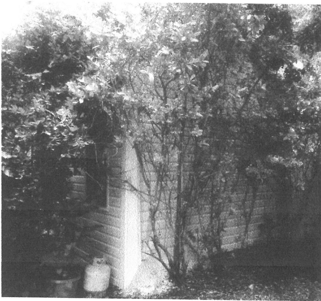
913 WHITE STREET ACCESSORY STRUCTURE VIEW FROM SOUTHWEST
