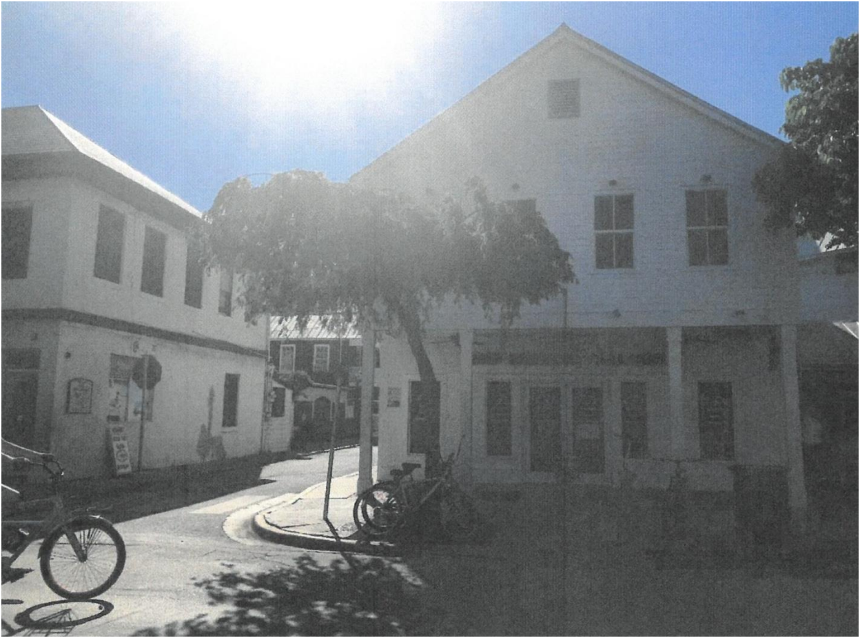
Right Neighboring Building Photograph.
