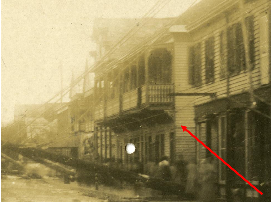
Historic photo from 1909 showing 210-216 Duval with wood lap siding and three second-story porches facing Duval.
