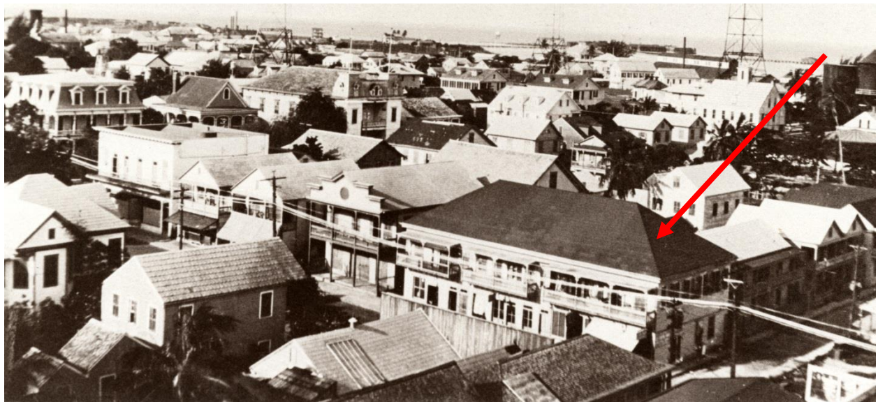
Historic aerial photo (undated). 210-216 Duval indicated by red arrow.
