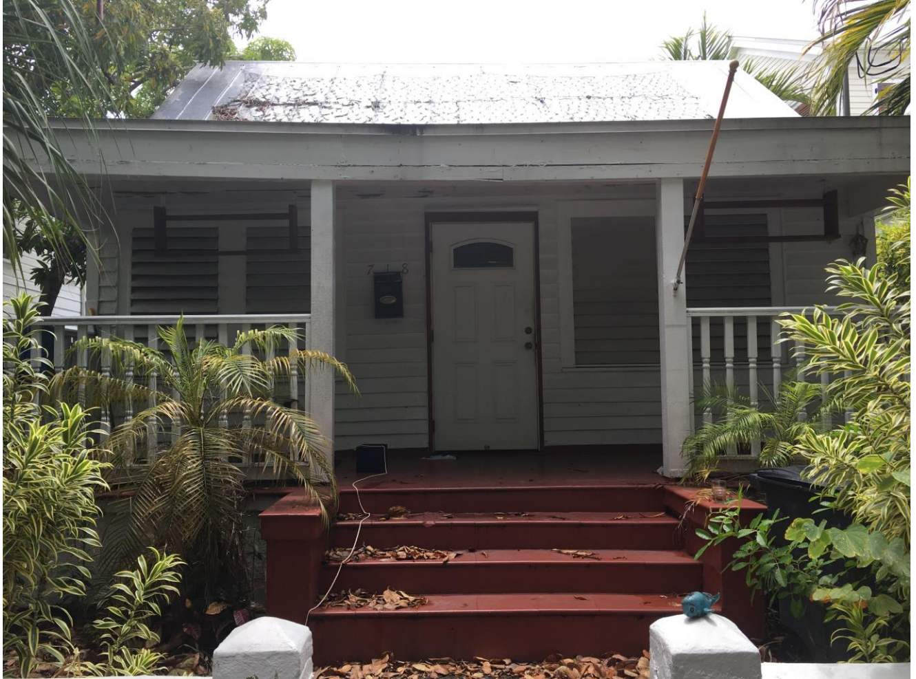
718 Windsor Lane Front entrance
