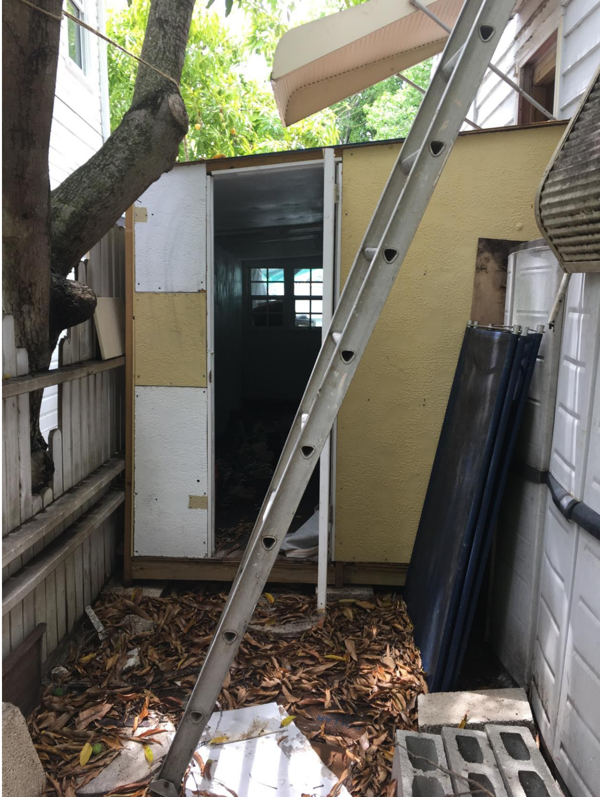
Side structure to be removed.
