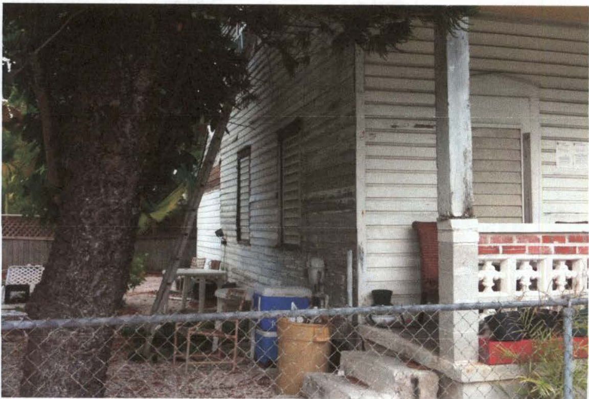
STREET SIDE FACADE
