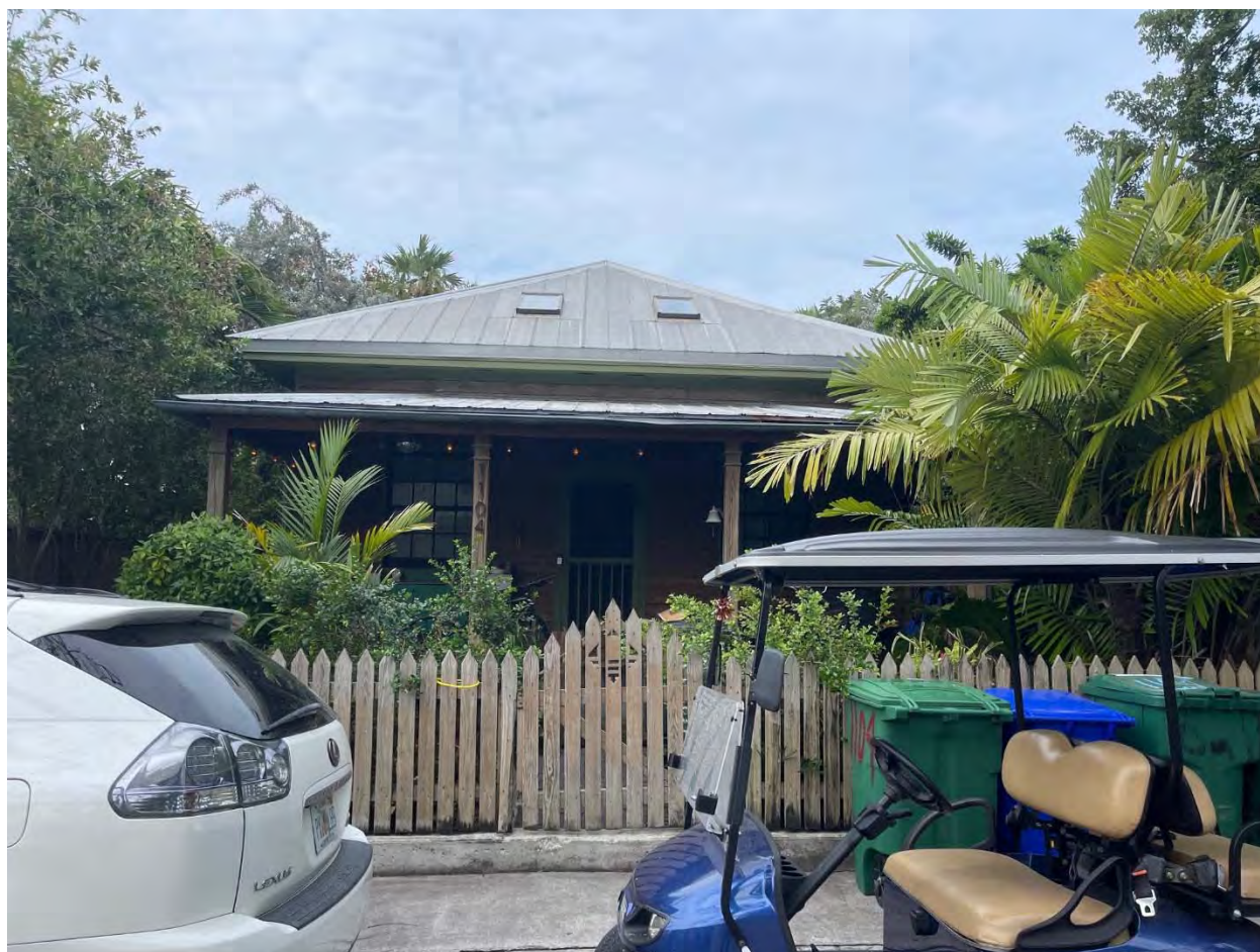
Façade / Street View
