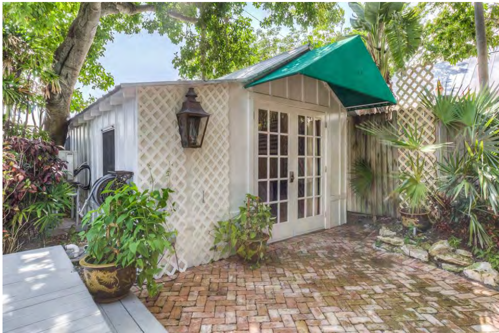
The only adjacent accessory structure to the property that staff was able to find is this one-story frame structure at 1100 Margaret Street.
