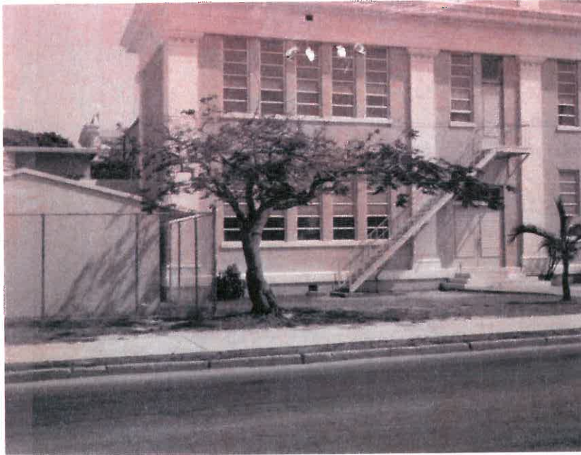
This photo of the United Street façade of Building B was taken in 1970. The auditorium can be seen at left. The shed in the foreground at left has been removed.
