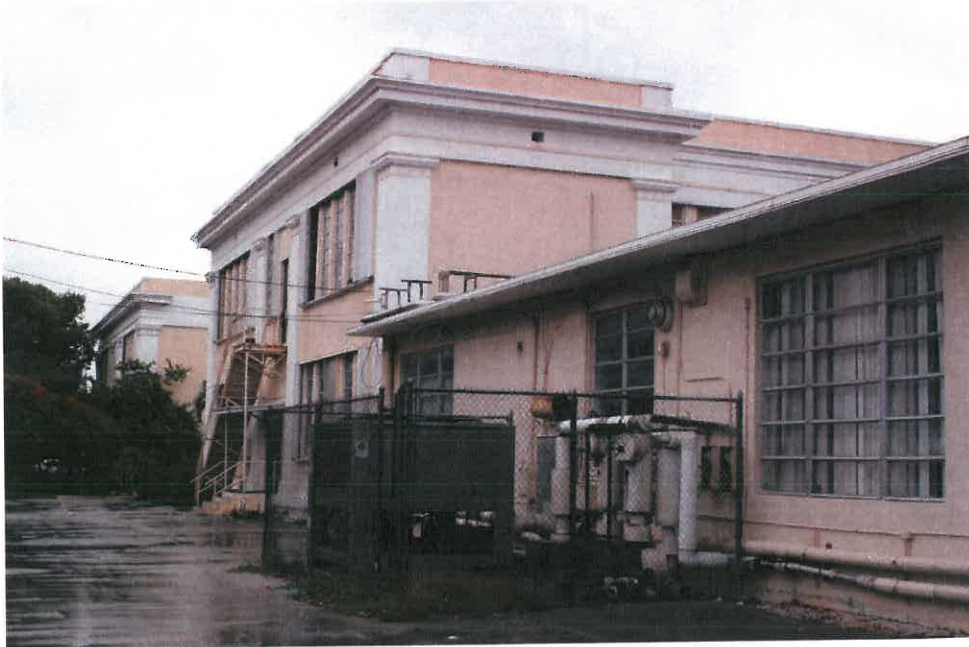
North elevation of Buildings B and C. Building C was removed in Spring 2014.
