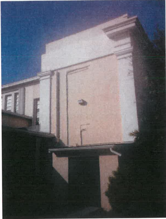
Building A, west façade.
