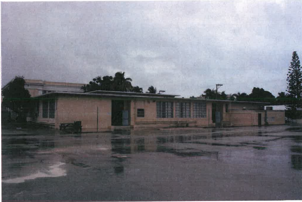
Building C, rear (west) elevation. Building C was removed in Spring 2014.
