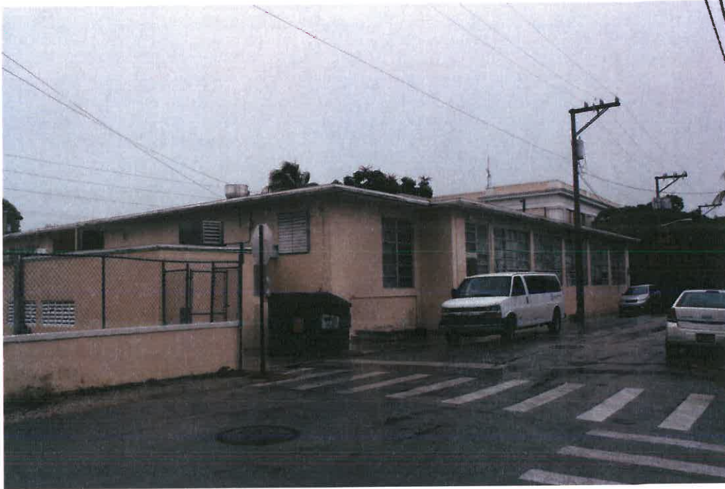
Building 'C', south elevation along Seminary Street. This building was removed in Spring 2014.
