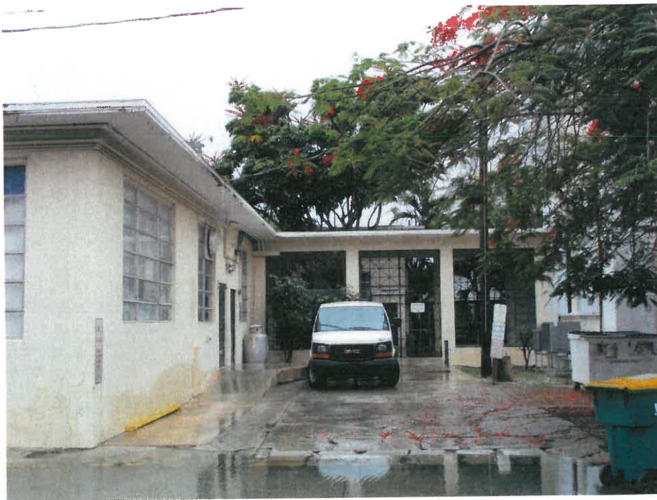
Building C, east façade, showing loading area along Seminary Street. Both Building C and the covered walkway are being removed in Spring 2014. Building B, at left, shall remain.
